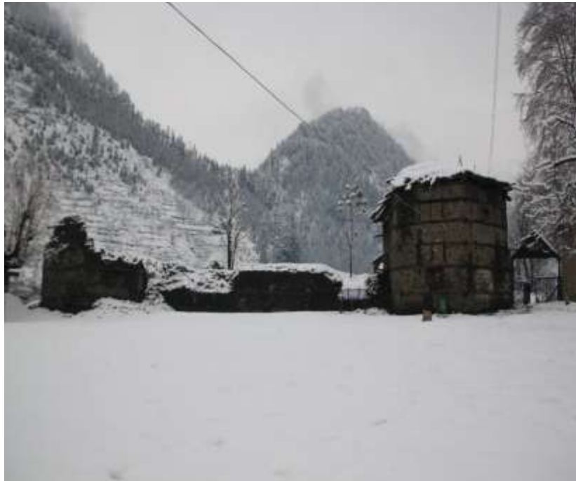
Fig. 67: A general view of Dogra fort Sharda, Neelum Valley
