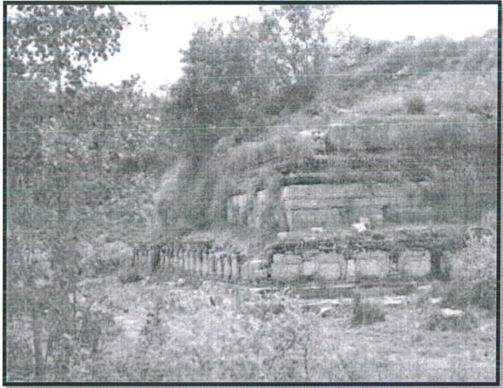
Figure 27: View of Kunala Stupa base and plinth
