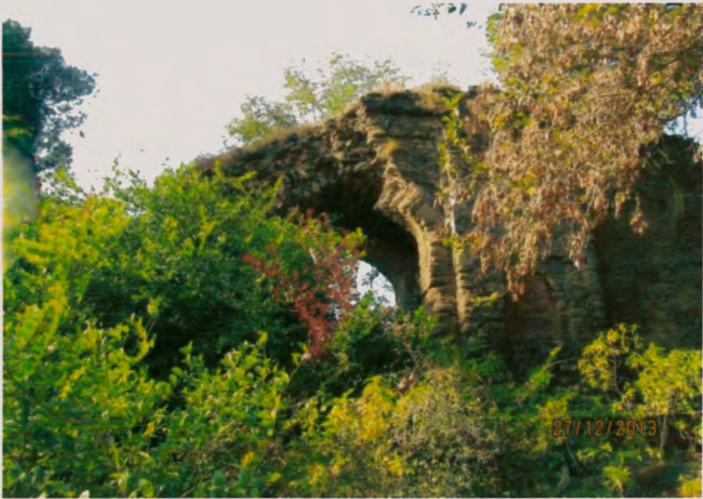
Figure 71 Façade of Ziarat Gate.
