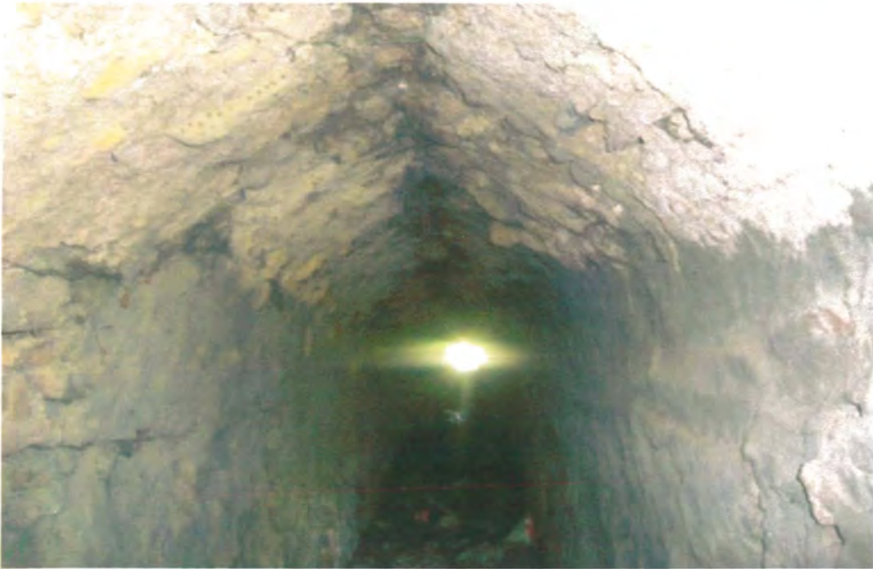
Figure 25 An internal view of the Tunnel of Sar Jalal
