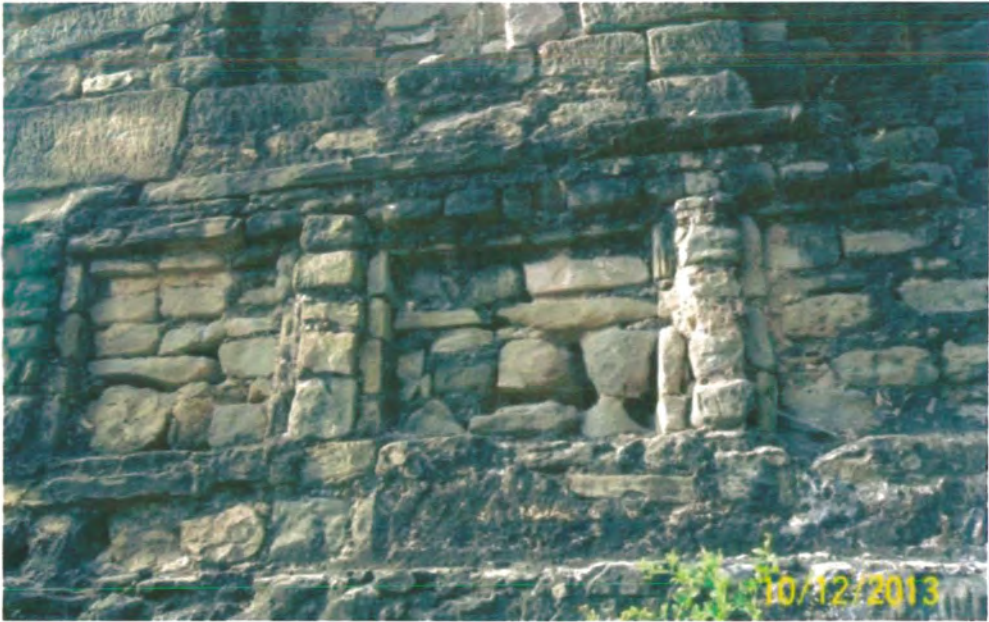
Figure 64 Blind panels at the base of Hathi Gate.
