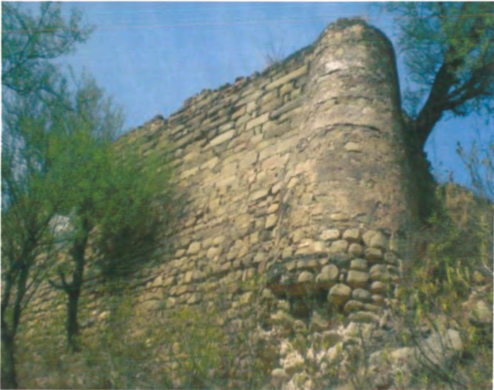
Figure 14 Bastion and the fortification wall of Dangali fortress
