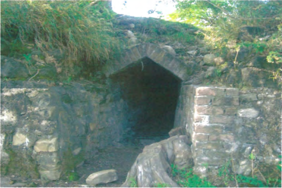
Figure 24 External view of the Tunnel of SarJalal.
