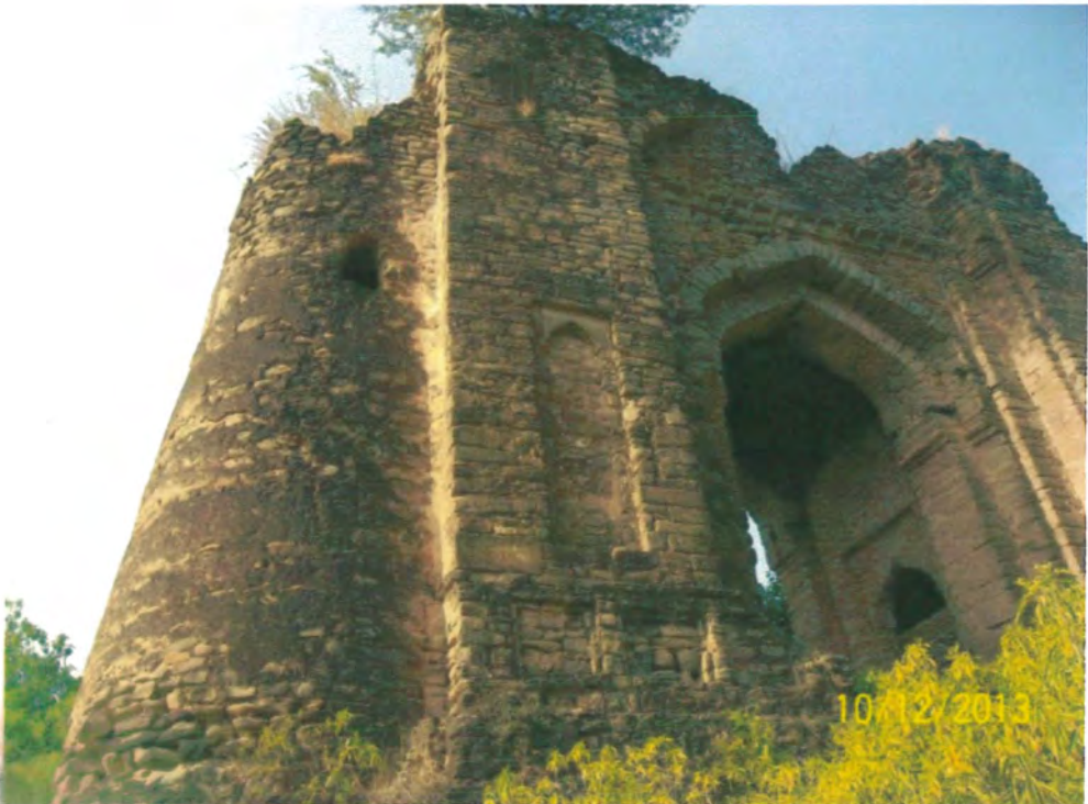
Figure 63 Frontal view of Hathi Gate.
