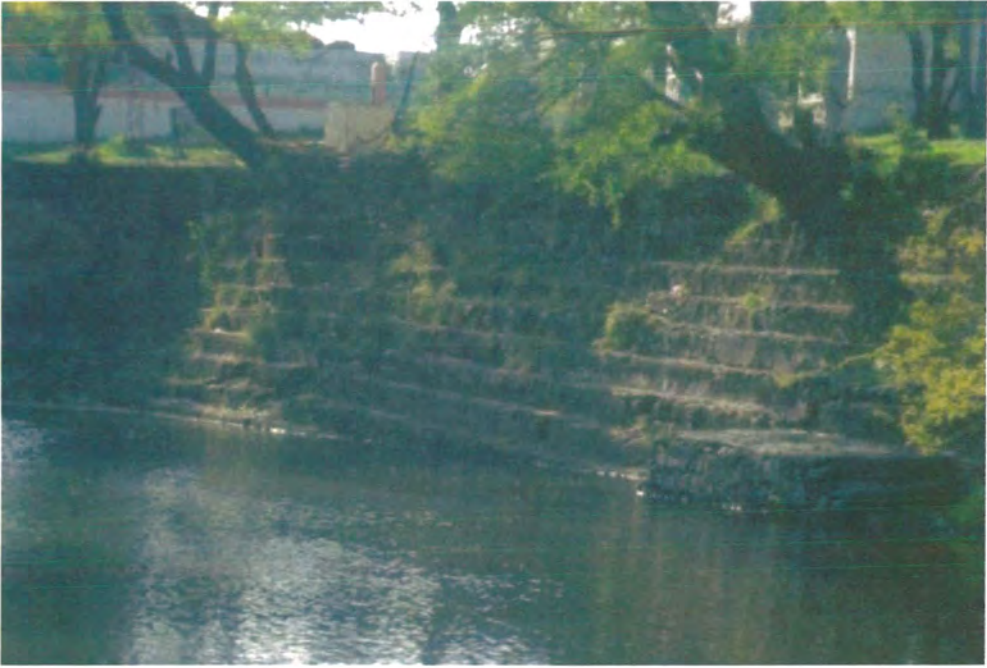
Figure 20 Another view of the Sar Jalal water tank.
