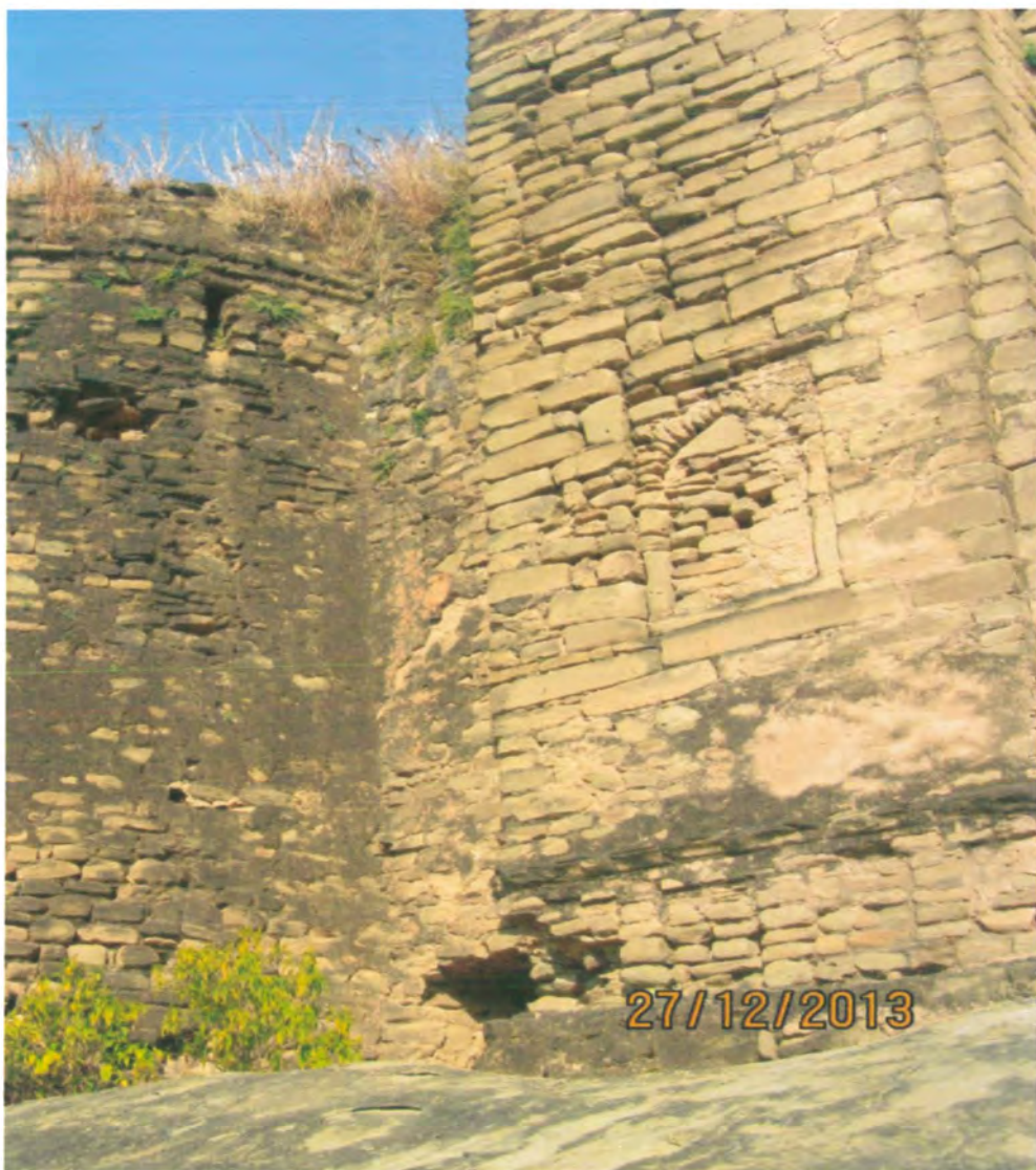
Figure 56 False arch niche at front of Lashkari Gate.
