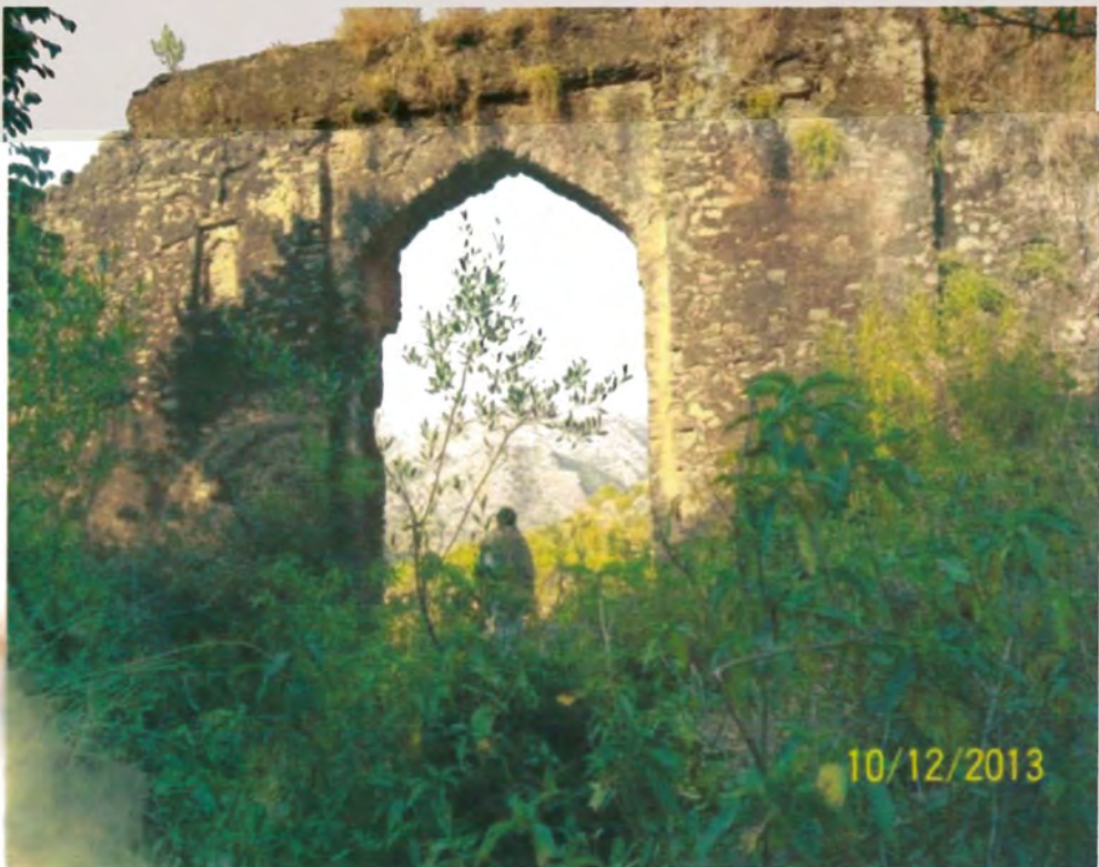
Figure 72 An internal view of Ziarat Gate.
