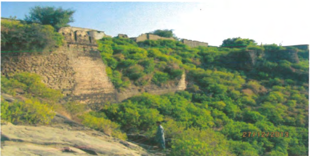
Figure 41 Fortification wall with battlement.
