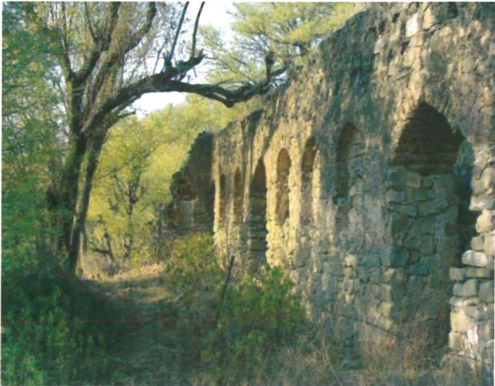
Figure 13 General view of Dangali Fortress
