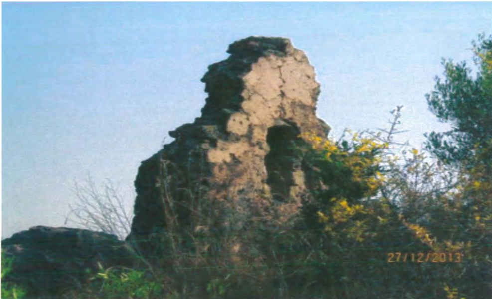
Figure 38 A view of Merlon and Slit of Pharwala Fort.
