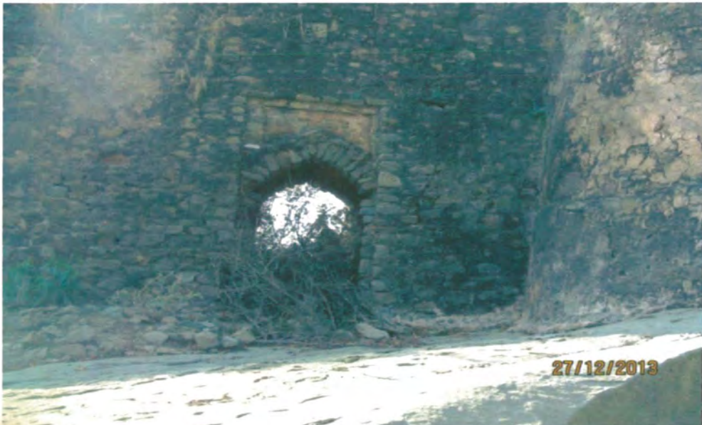
Figure 79 Façade of Escape Gate.
