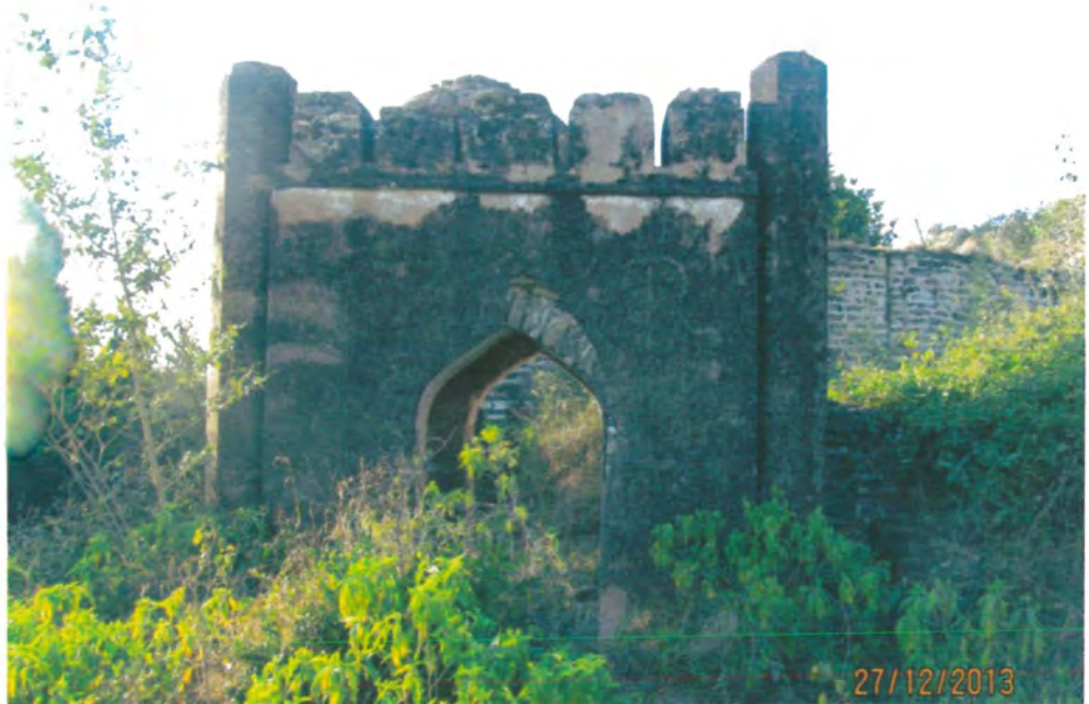
Figure 84 Front view of the vestibule.
