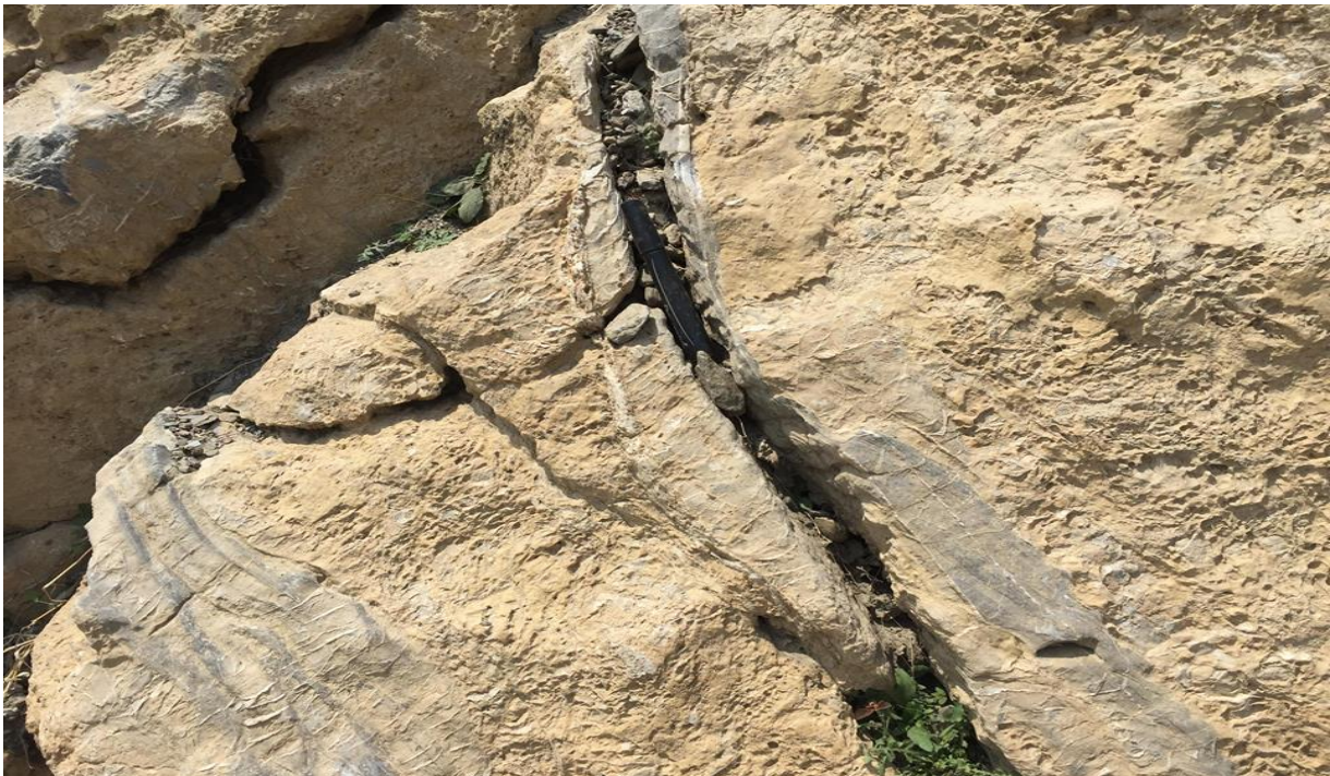
Fig 4.5 Highly fractured, jointed, porous limestone, showing vuggy porosity. Algal stromatolites are also visible in the picture. This is the unaltered limestone away from the dyke.
