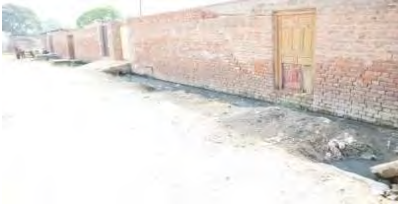
Figure 9 View of sewage system in the village
