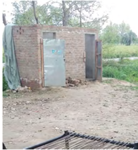
Figure 11: Recently constructed washrooms for the visitors
