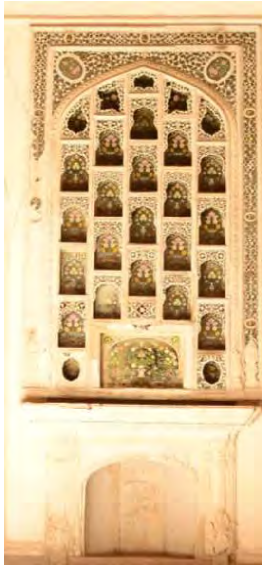
Fig. 6. 3. Cheeni khana above a fire place in the center of a room. Photograph by researcher
