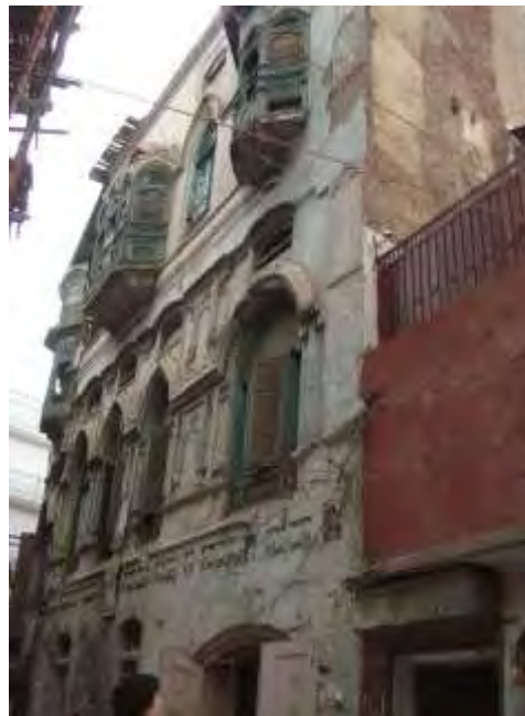
Fig. 2. 4 A View of Raj Kapoor haveli. Photo by researcher 2015
