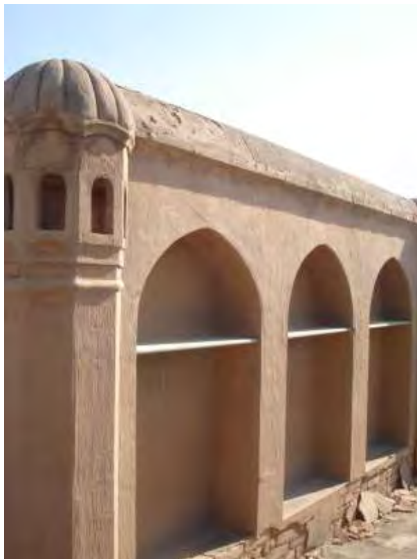
Fig. 4.57. Boundary wall on north. Photo by researcher
