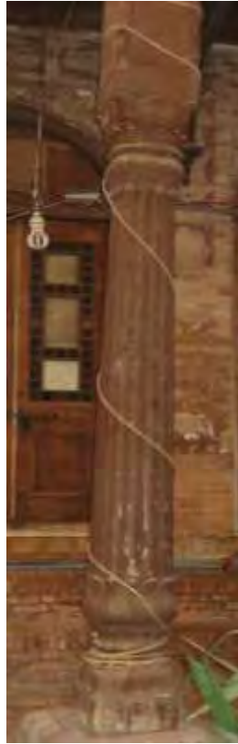
Fig. 2. 19. Detail of a pillar. Photo by author.
