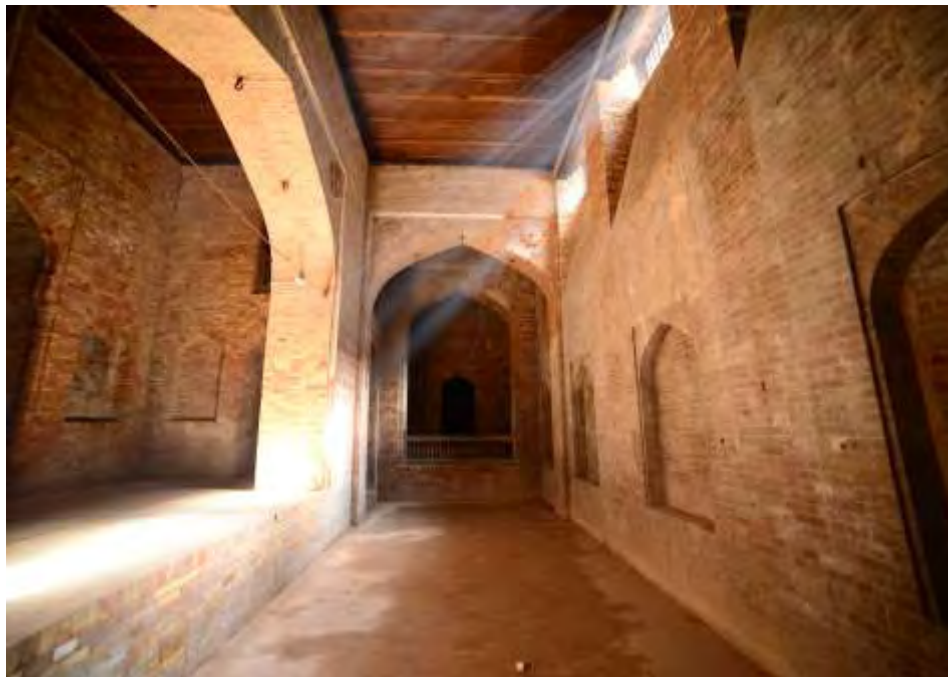
Fig.4 .38 view of windows opening in the central courtyard. Photo by researcher
