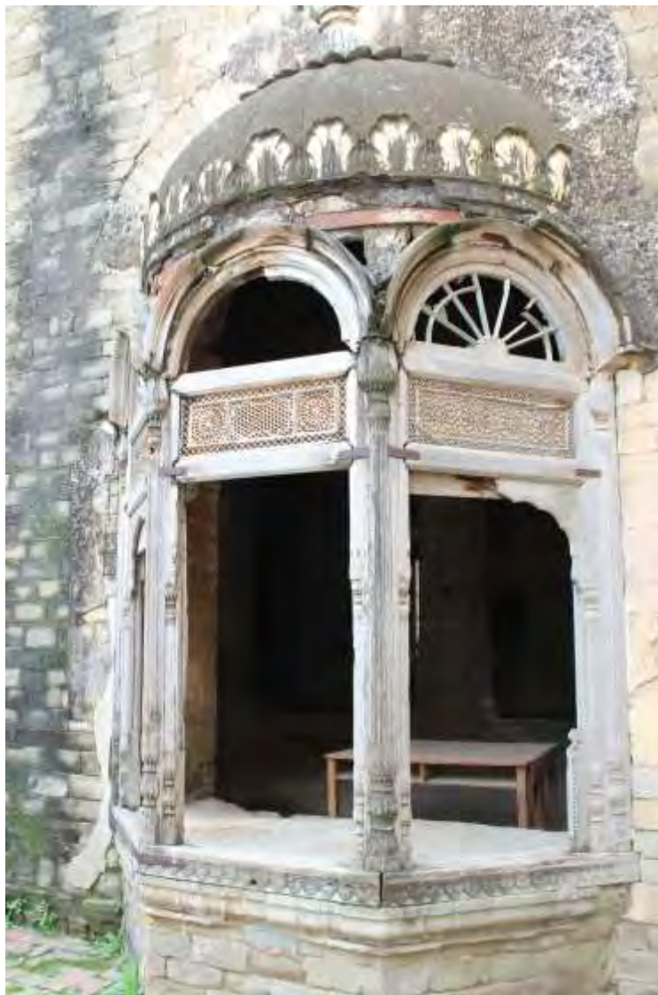
Fig. 6. 17. Window Jharoka in Khem Bedi Sigh haveli Kallar Sayedan. Photo by author
