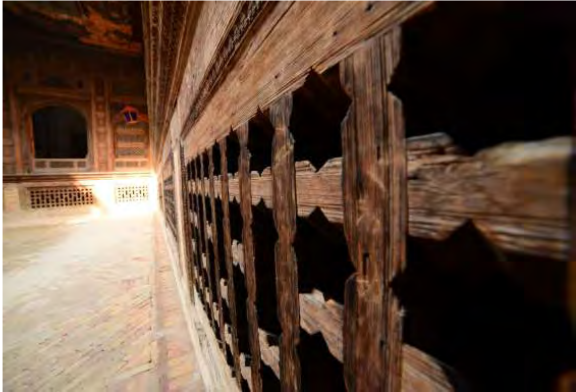
Fig. 5. 25 Jali Screen or ventilators. Photograph by researcher
