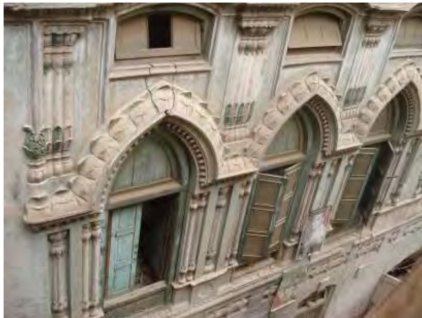
Fig. 2. 7. Outer view of Raj Kapoor haveli . Photograph by researcher Dec 2015
