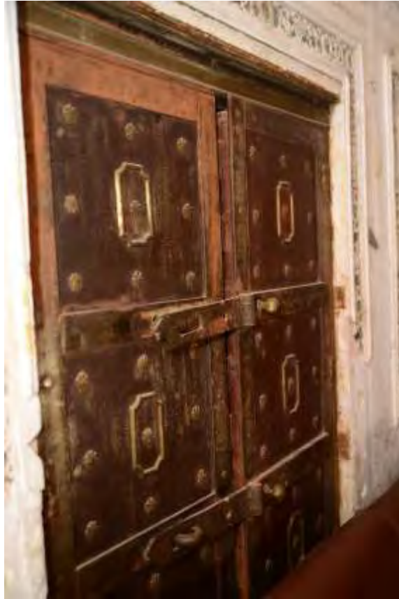
Fig.4 .27. A safe in northern room. Photo by Author
