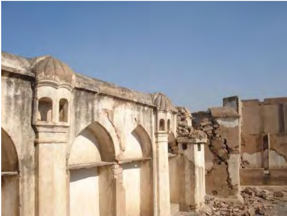
Fig.4 .58 View of the wall with demolished areas. Photo by researcher
