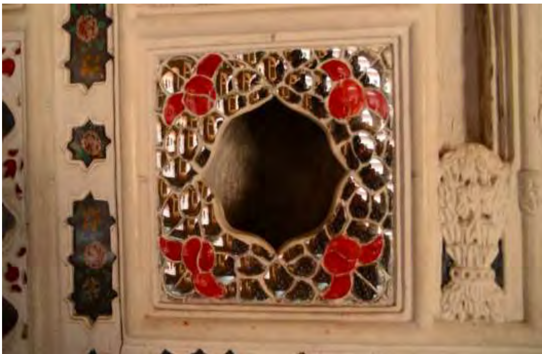
Fig. 6 .2. Detail of Gilded stucco and mirror work on Cheeni khan. Photo by researcher
