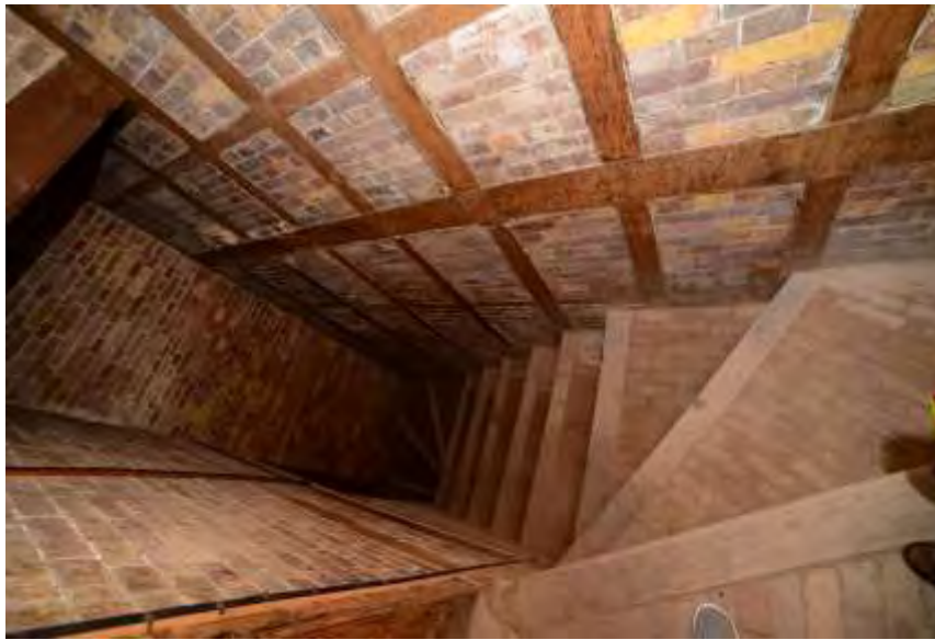
Fig.4 .34 Stairs going to the basement. Photo by researcher
