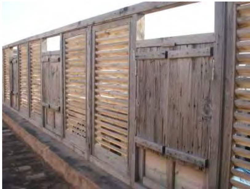
Fig. 4.55 view of the wooden fence. Photo by author
