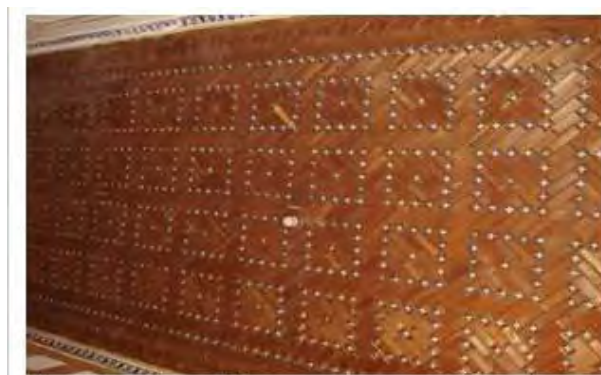
Fig. 5. 8 Another ceiling room 7 of ground floor photograph by researcher
