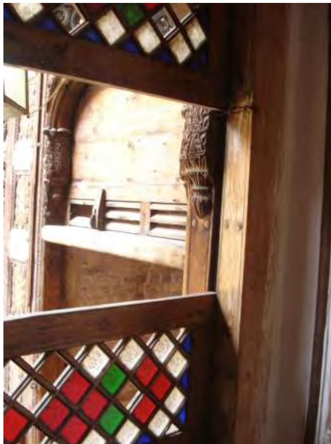
Fig. 4.6. View of stain glass window from north bala khana. Photo by author
