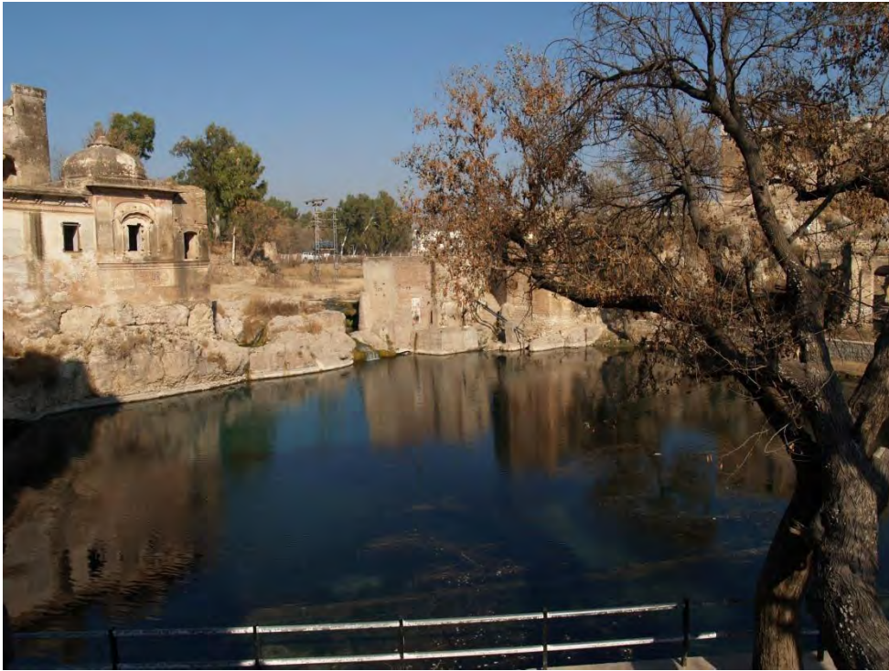
Figure 5 Katas Raj Temples Pond prior to Conservation (Photo Courtesy Dr. Ilyas Bhatti)
