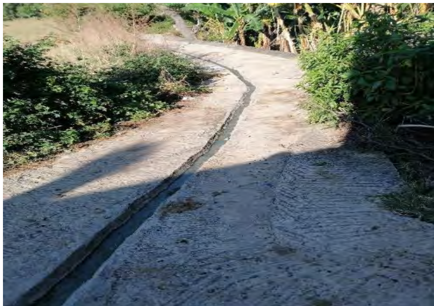
Figure 14: Street with sanitation channel
