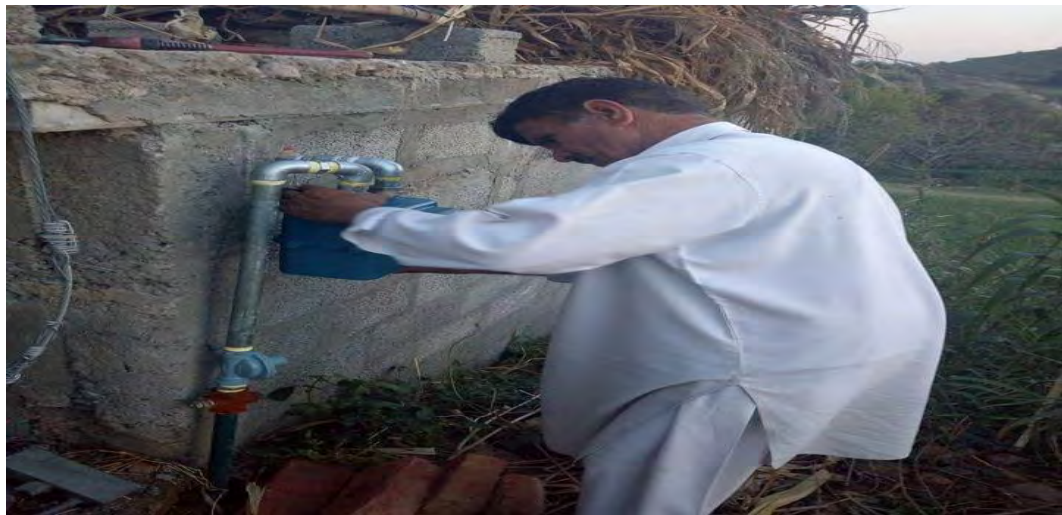
Figure 10: Gas meter being installed
