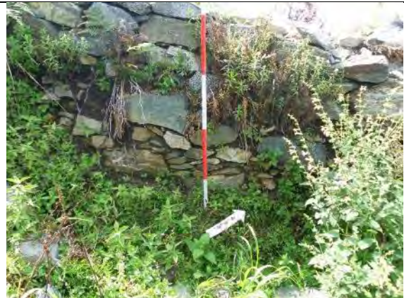
Fig. 6. Picture shows recent construction over old structure
