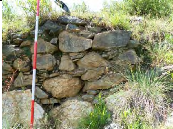
Fig. 10 walls portion of disturbed diaper masonry
