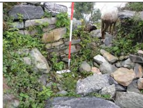
Fig. 8. The upper part of the wall shows recent activities and the lower part with pure diaper masonry is the evidences of Buddhist period
