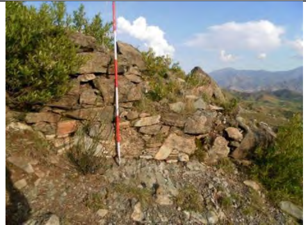
Fig. 2. Stone structure with rough semi-diaper masonry
