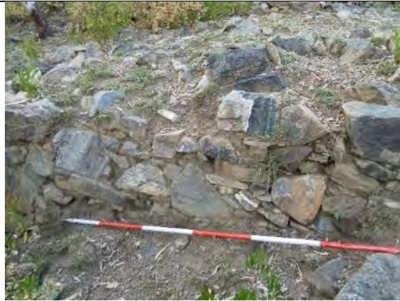
Fig. 2 wall portion with ranging rod
