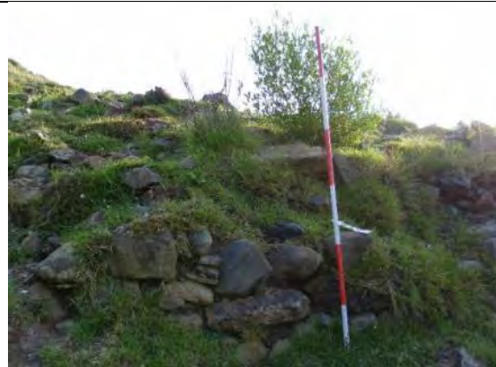
Fig. 2. Signs of wall
