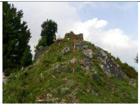
Fig. 14. A packet made by the army using stones of the old construction
