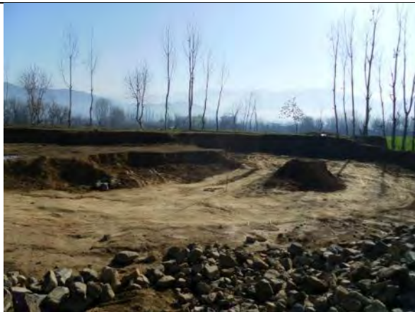
Fig. 3. Whole view of the site
