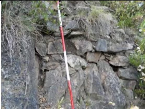
Fig. 5 Wall portion with ranging rod
