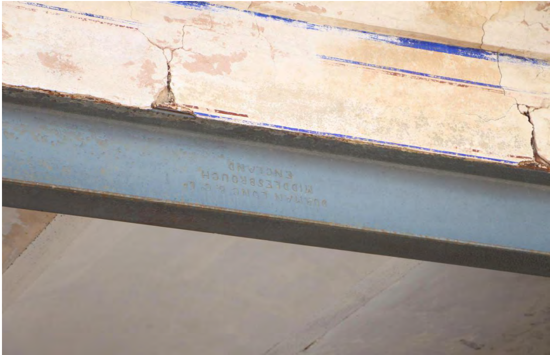
Plate 43 Iron lintel supporting the roof (Photo taken by Researcher)
