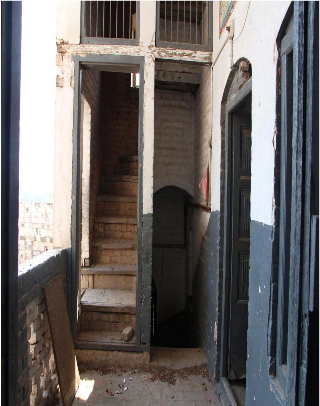
Plate 47 Stairs for top floor (Photo taken by Researcher)
