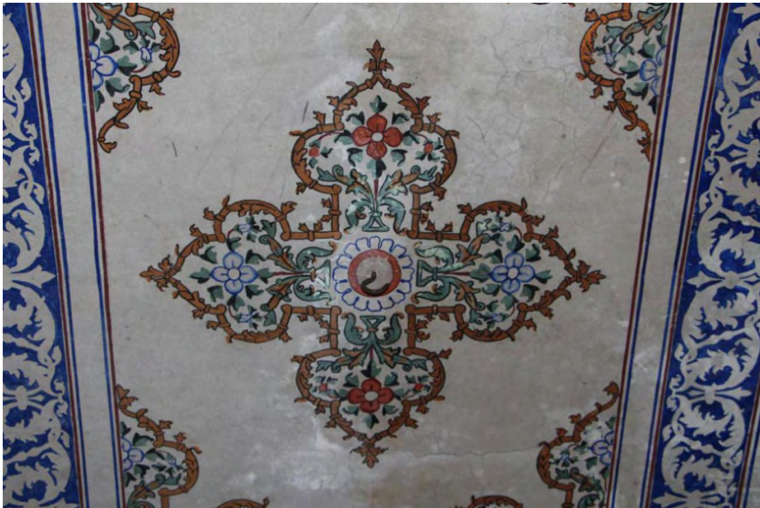
Plate 91 Detail of a roof panel (Photo taken by Researcher)
