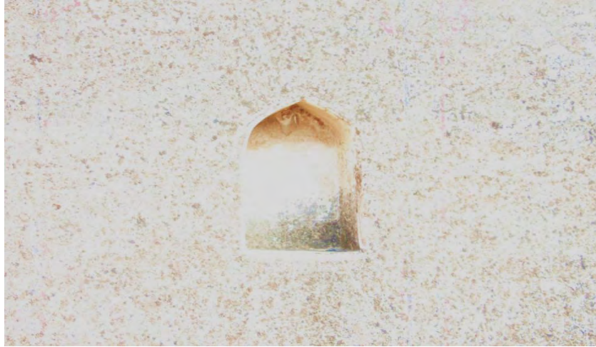
Plate 7 Arched niches on top floor wall (Photo taken by Researcher)
