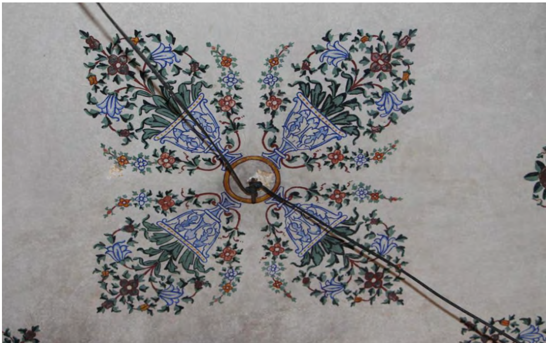
Plate 99 A roof panel showing arrangement of four pots, filled with floral stems and acanthus leaves.
