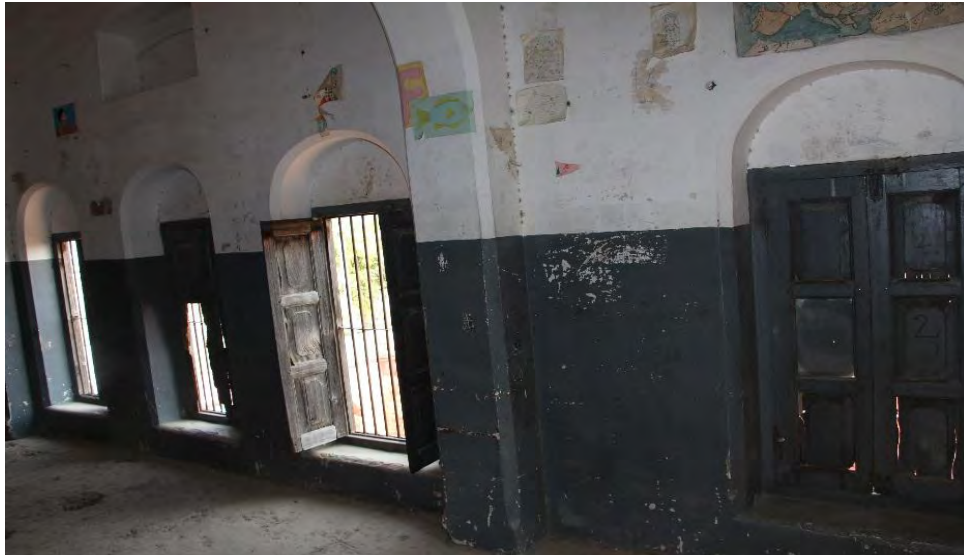
Plate 18 Windows in a row on first floor (Photo taken by Researcher)
