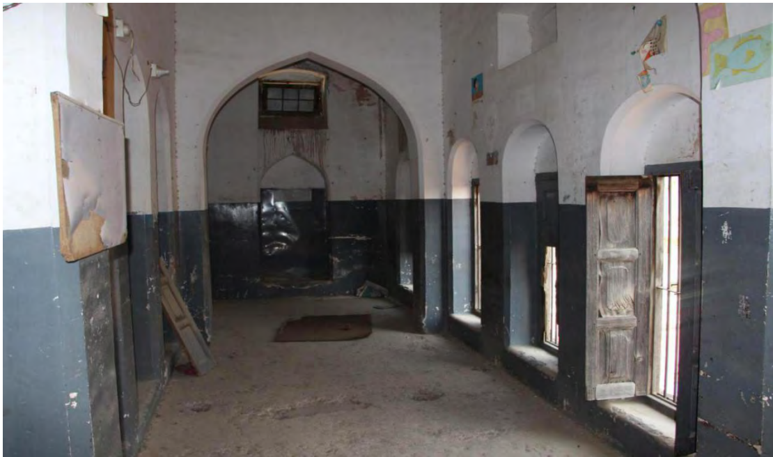
Plate 44 interior of first floor (Photo taken by Researcher)
