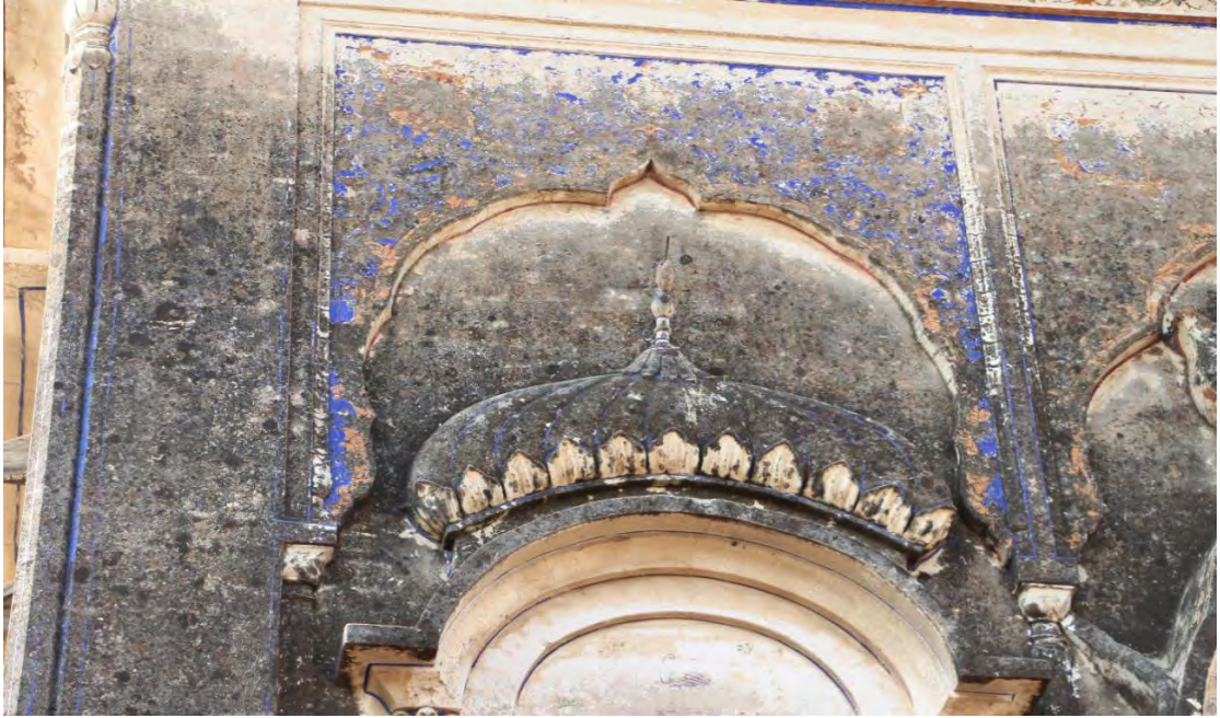
Plate 11 Multi cusped blind arch with dome in relief form (Photo taken by Researcher)
