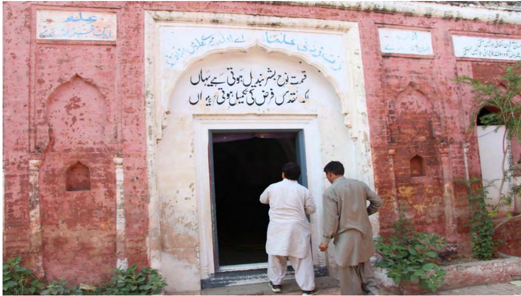
Plate 30 A view of the facade (ground floor) (Photo taken by Researcher)
