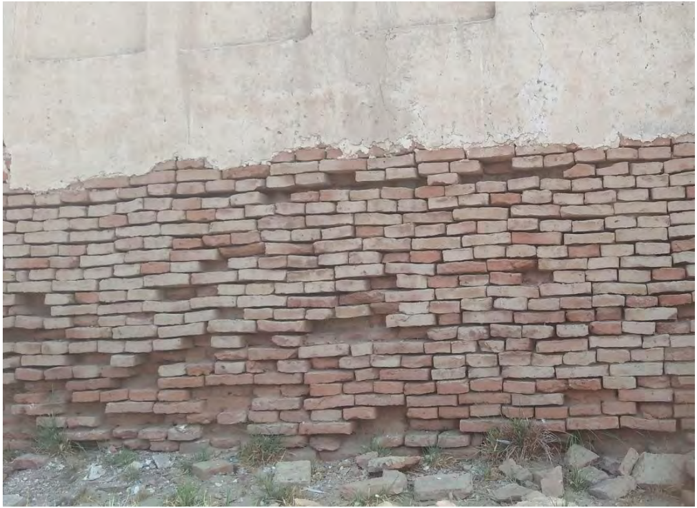
Plate XVI: Naked brick masonry border on exterior of the building (photo by researcher)
