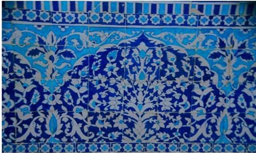
Plate I: Kashi Tiles found at Sachal Sarmast Dome
