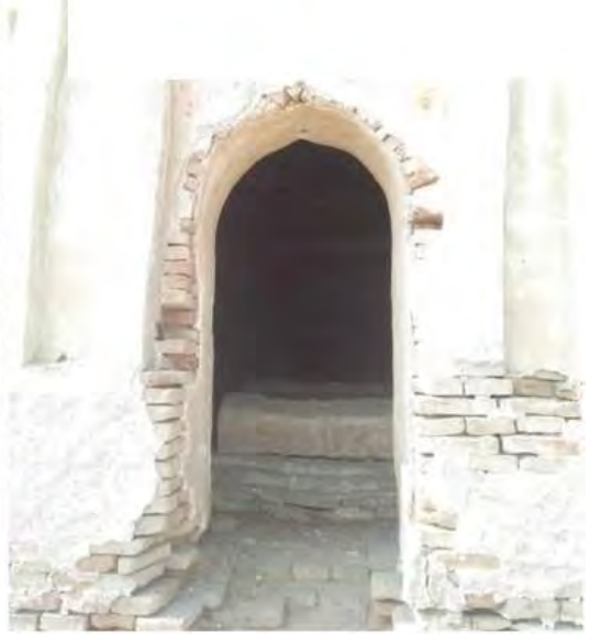
Plate VI: Pointed Arch of Main Entrance (photo by Researcher)
