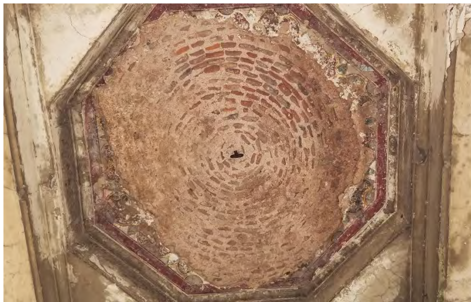
Plate 26 Interior of Dome Shows Bricks used for Decoration (Photograph by Researcher)
