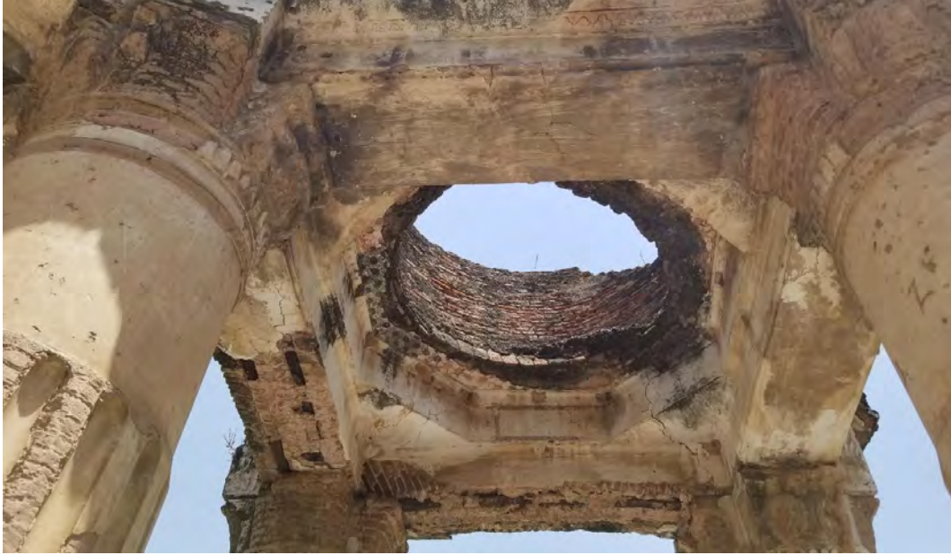
Plate 74 Demolish Structure of Southern Dome (Photograph by Researcher)
