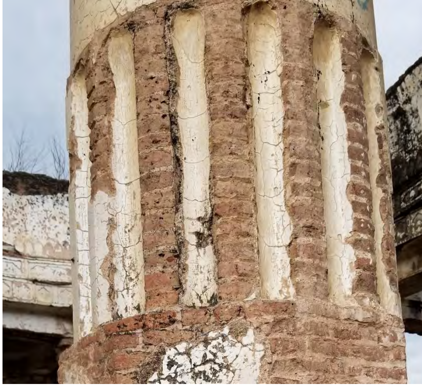
Plate 70 Flutes in Stambha or Column (Photograph by Researcher)
