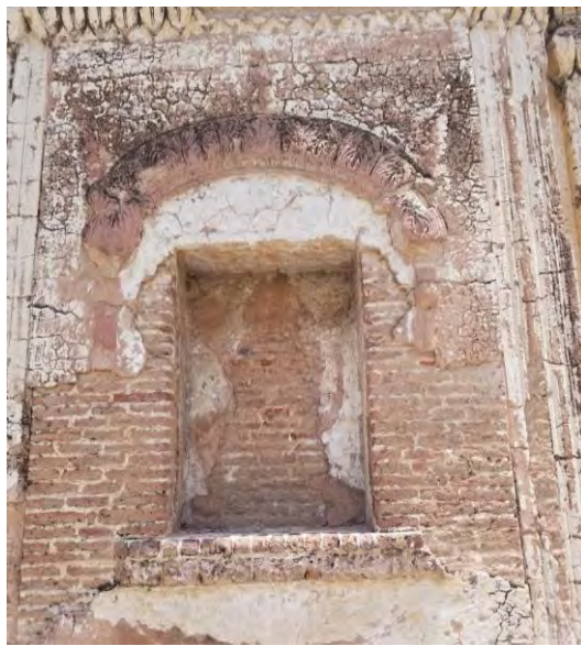
Plate 55 Niche at Northern Side of Shikhara (Photograph by Researcher)
