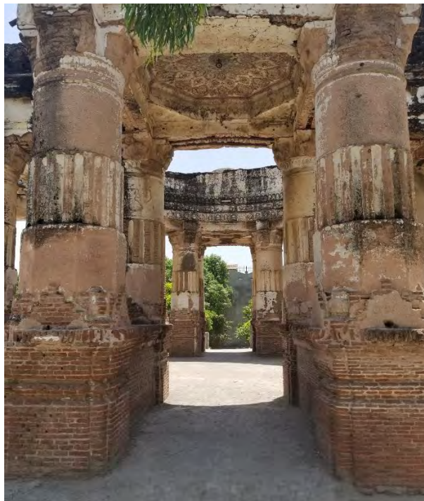
Plate 32 View of Western Colonnade Entrance Way (www.google.com)
