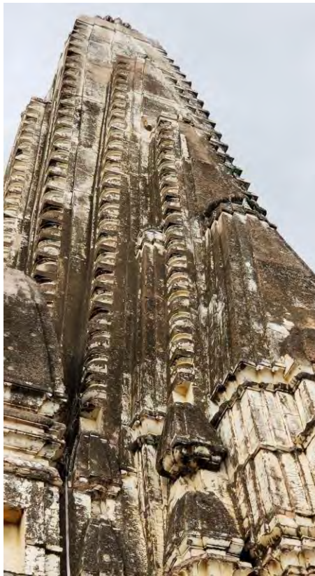
Plate 53 Northern View of Shikhara, representing recesses of Shikhara (Photograph by Researcher)
