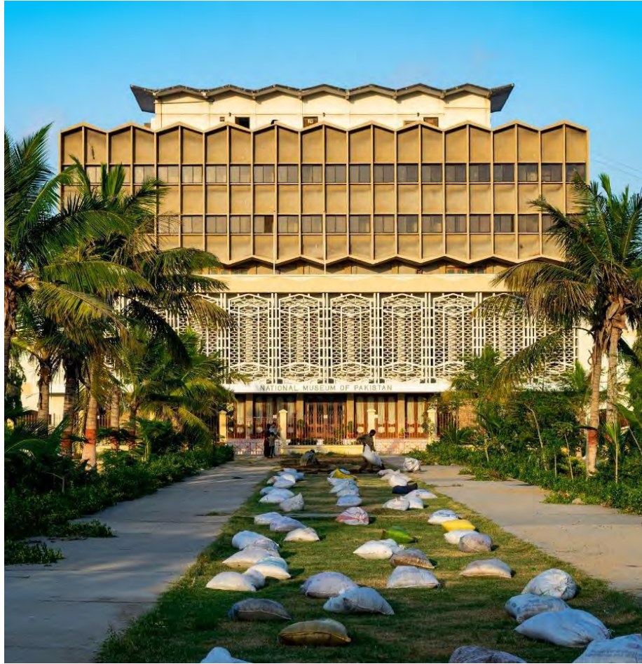
Fig. 2: Existing building of NMP, Karachi (Photo by Majid Karim)
