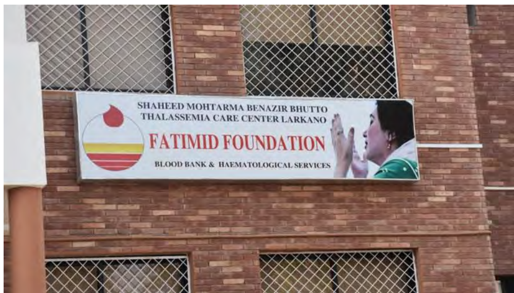
Figure 1: Source: field work
