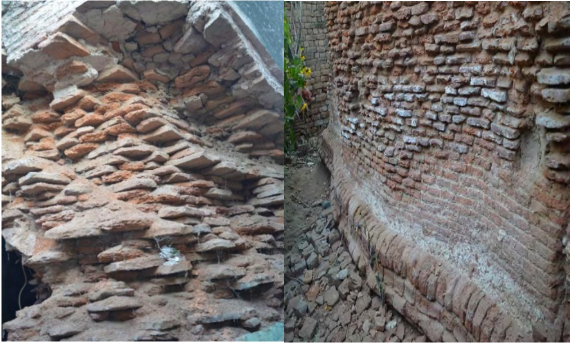
Figure 20 Material Used for Construction
