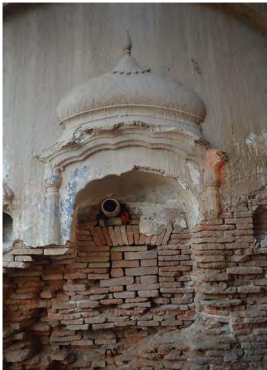
Figure 26 Decorative arches inside the chamber
