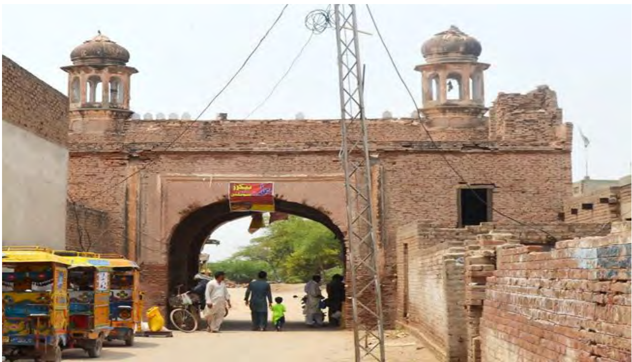
Figure 14 Back view of Kabulee Gate
