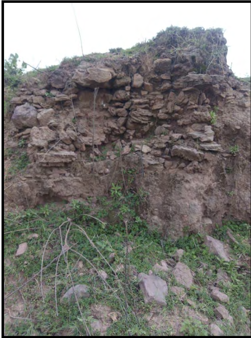
Figure 20: Wall remains. (Picture taken by the researcher)
