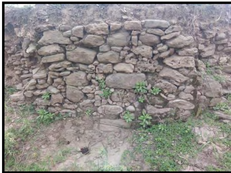
Figure 14: Wall Structure. (Picture taken by the researcher)
