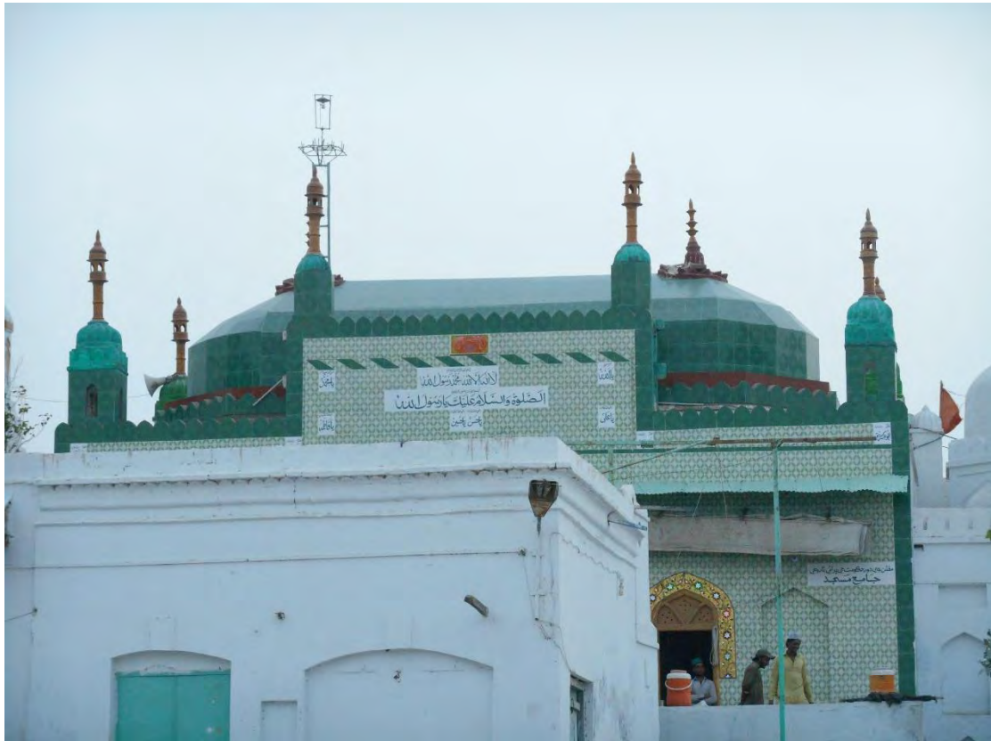
Figure 34: Close front view of Mosque; white color was removed, and the green color was painted on the Mosque in 2014, loudspeakers minarets and Islamic inscriptions were fixed on the Mosque's main entrance gate that was not present before.
