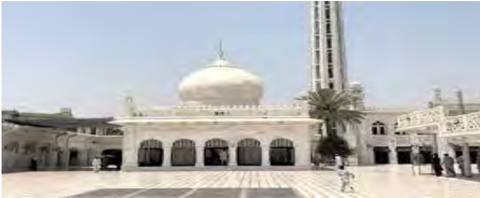
Figure 3. Source, Field Work
