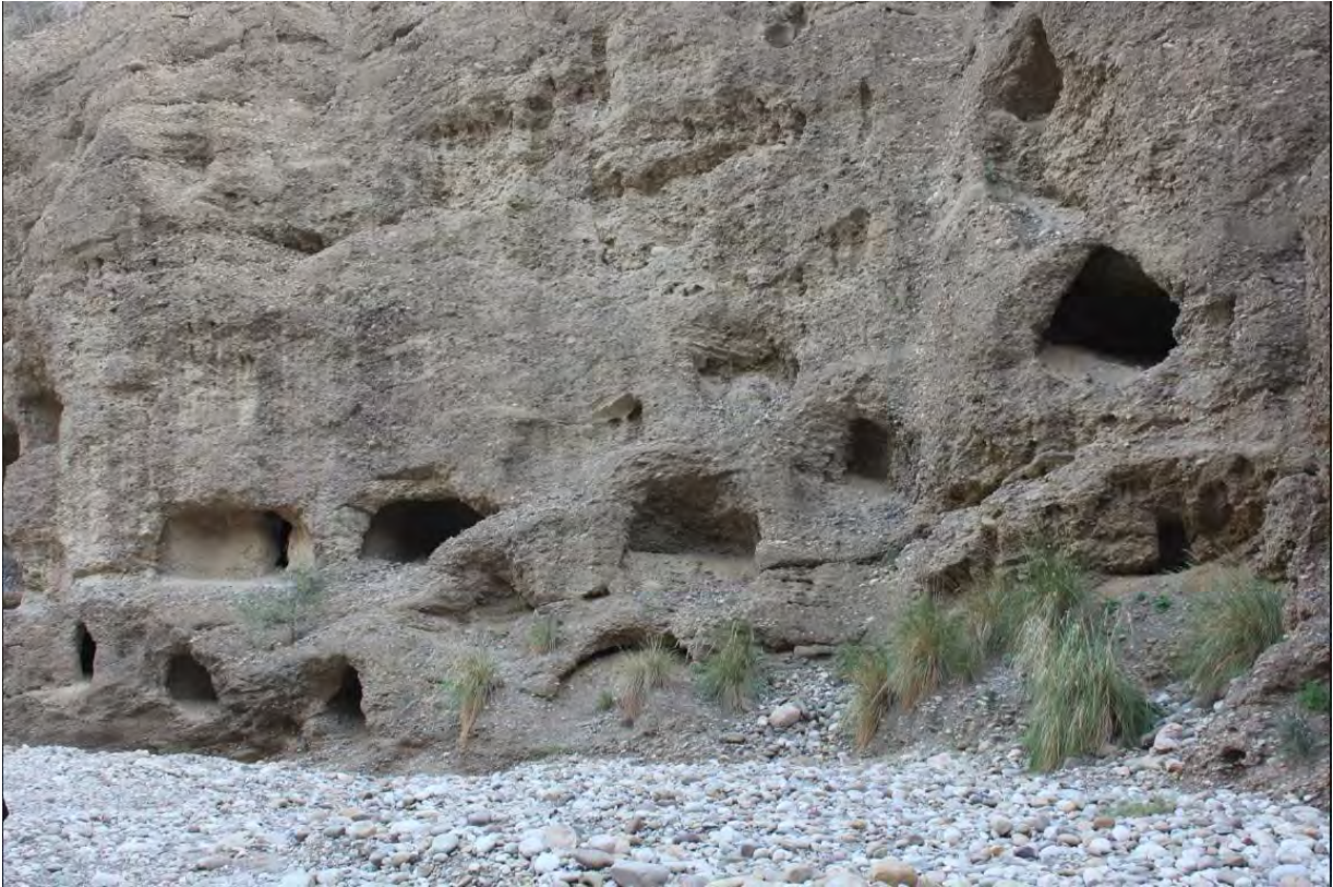
Fig 10: caves destroyed due to climatic conditions and flooding
