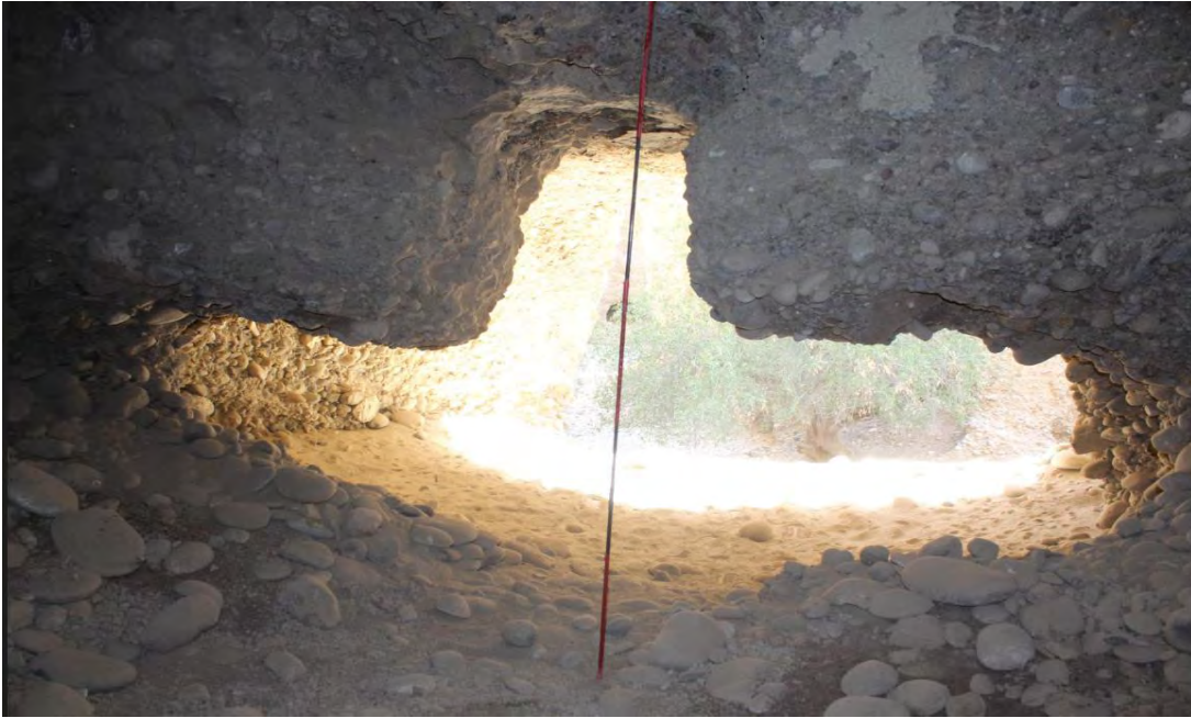
Fig 8: Inner portion of destroyed cave due to flooding
