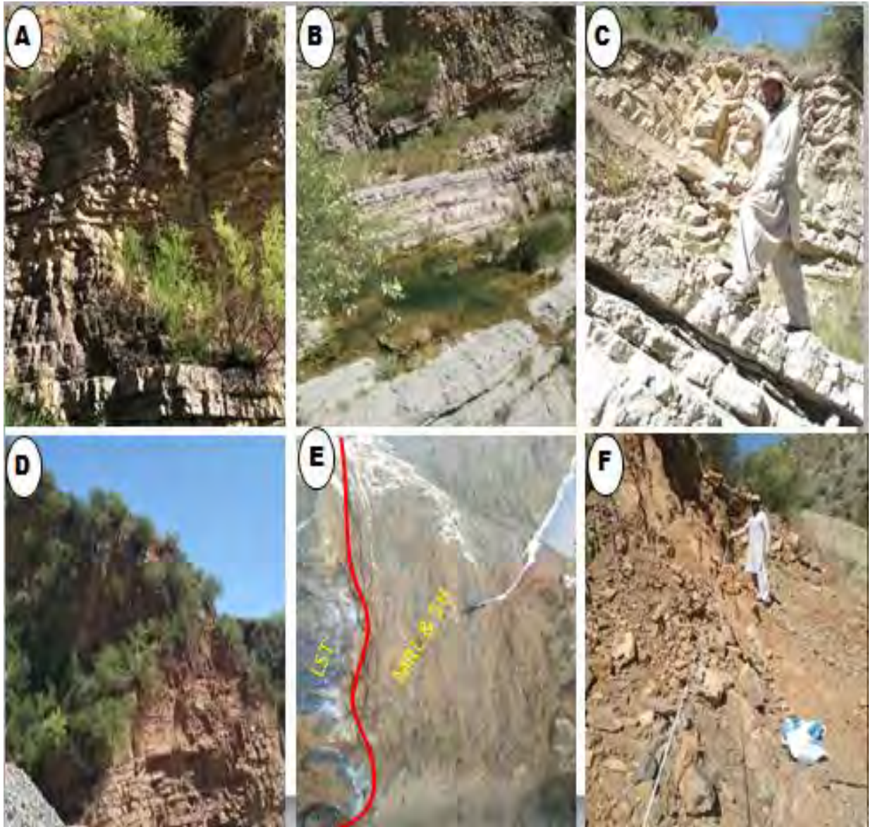
Figure 3.2 Field Photograph (A, B) shows fractures & solution weathering effect in limestone. (C) View of thick bedded limestone. (D) Shows interbedded shale and thin to medium bedded argillaceous limestone with vegetation cover. (E) Shows interbedded shale & marl with limestone. (F) Shows section measurement of Shinawari Formation in study area.
