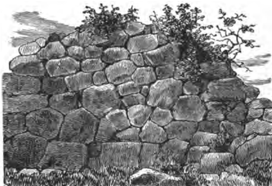
FIG. 51.—ANCIENT GREEK WALL OF UNWROUGHT STONE FROM SAMOTHRACE.
