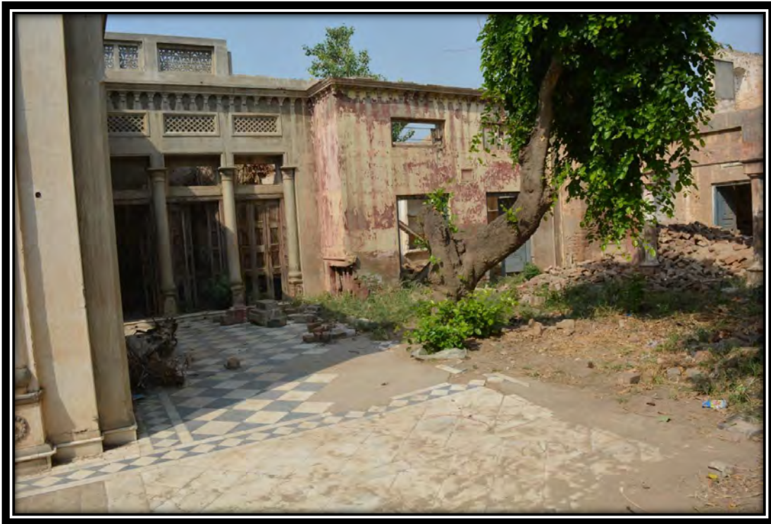
Figure 31: General view of the second hall and other ruins
