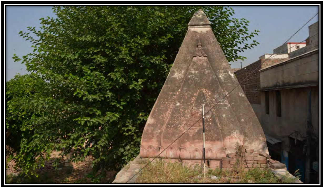
Figure 37: Upper view of the Sikhara of the Oam Mandir having the curvilinear structures
