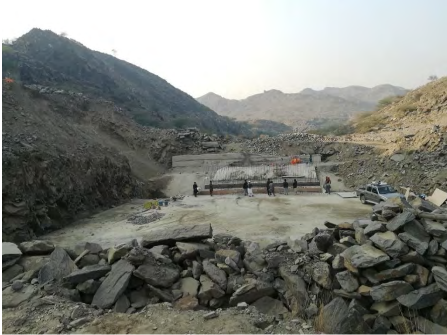
Figure 1.2: Jay Dam site
