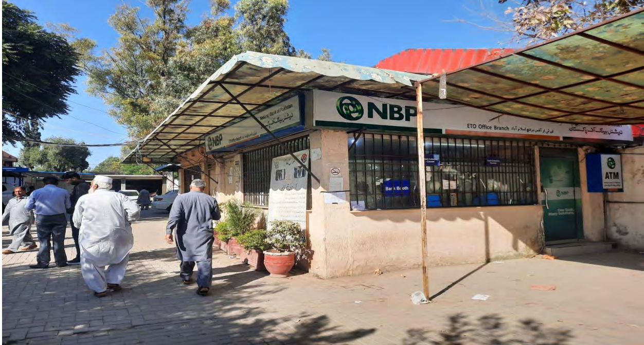
Figure 7, A branch of National Bank Pakistan in side of Excise office
