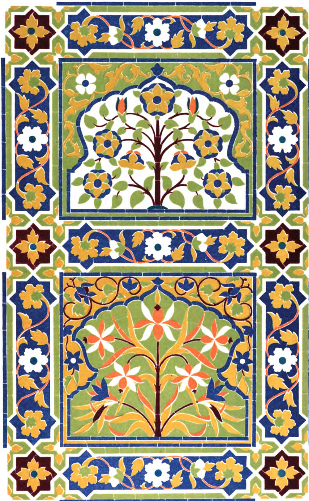
AGRA : CHINI-KA-RAUZA. TILED PANELS ON THE NORTH FAÇADE, EAST SIDE. Marked C, C, on the Elevation, Plate XXIV..
