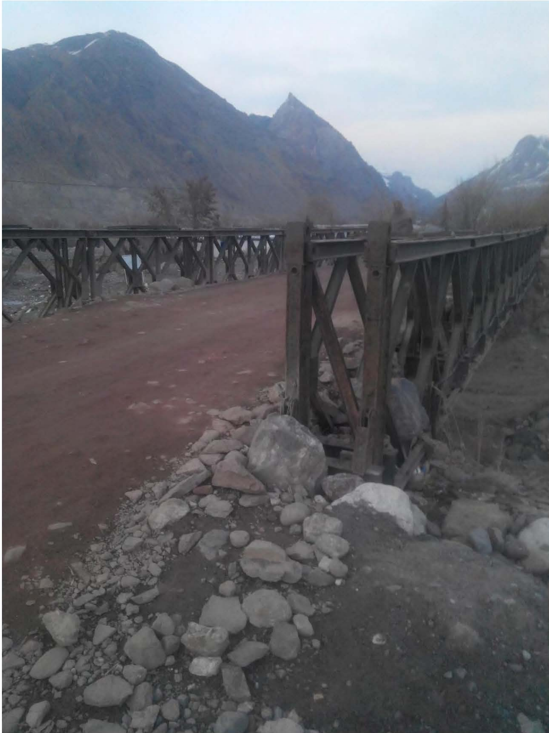
Photo 6.1: Bridge on Reshum Stream Installed by FWO after the Departure of the Army Chief
