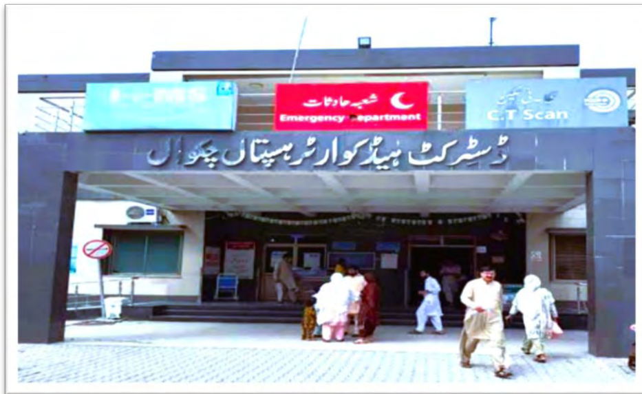
Figure-4 DHQ Hospital
