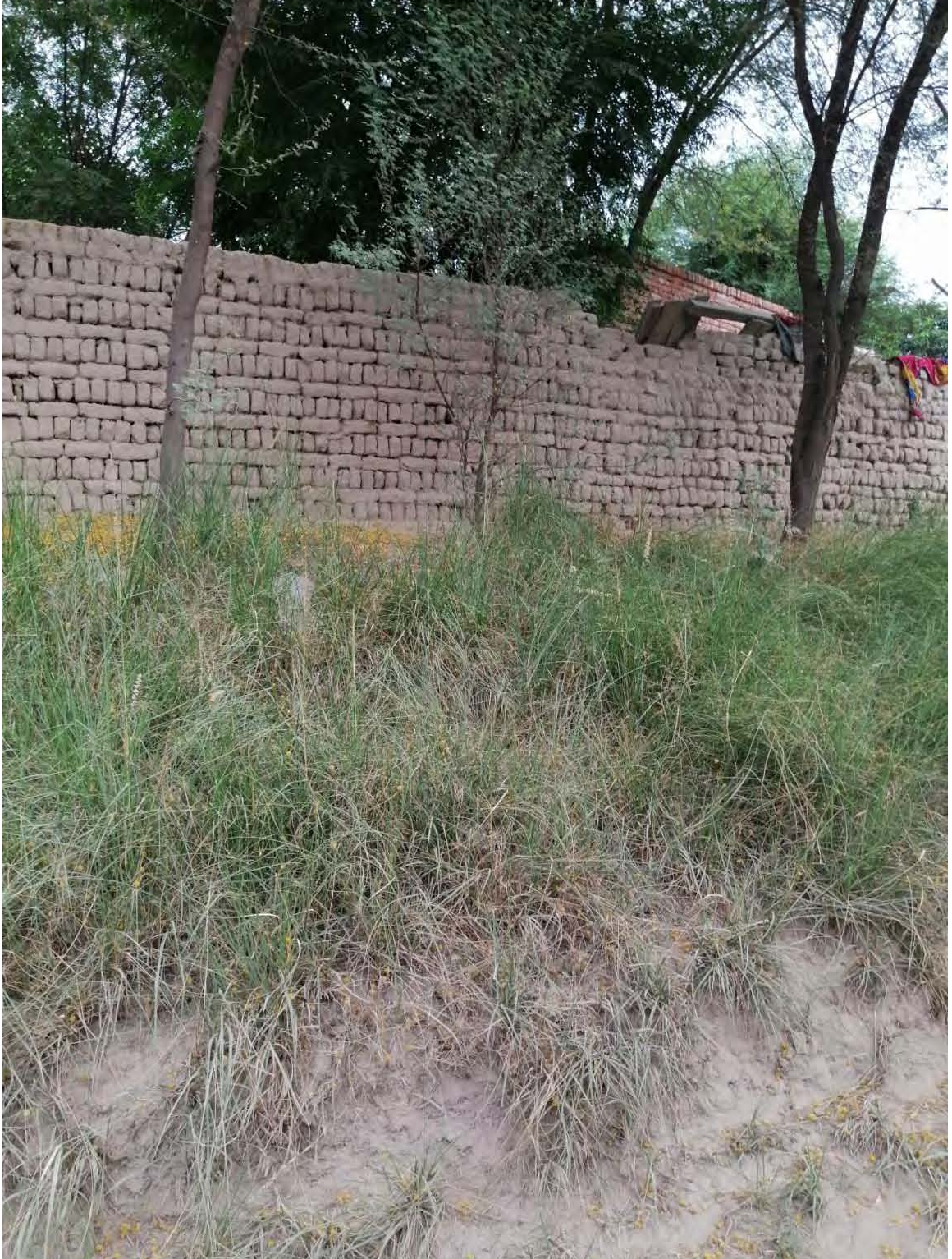
Each house is 8 to 12 feet higher from ground level.
