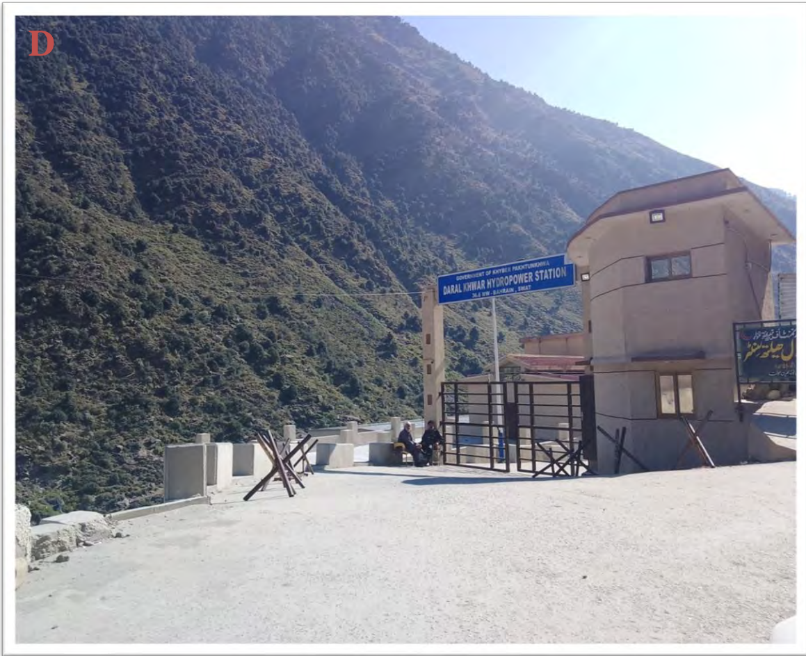
Figure 3.4 D showing Daral Hydropower also effected during 2022 flood and also the lower part of the project area is severely damaged and flown by the river.
