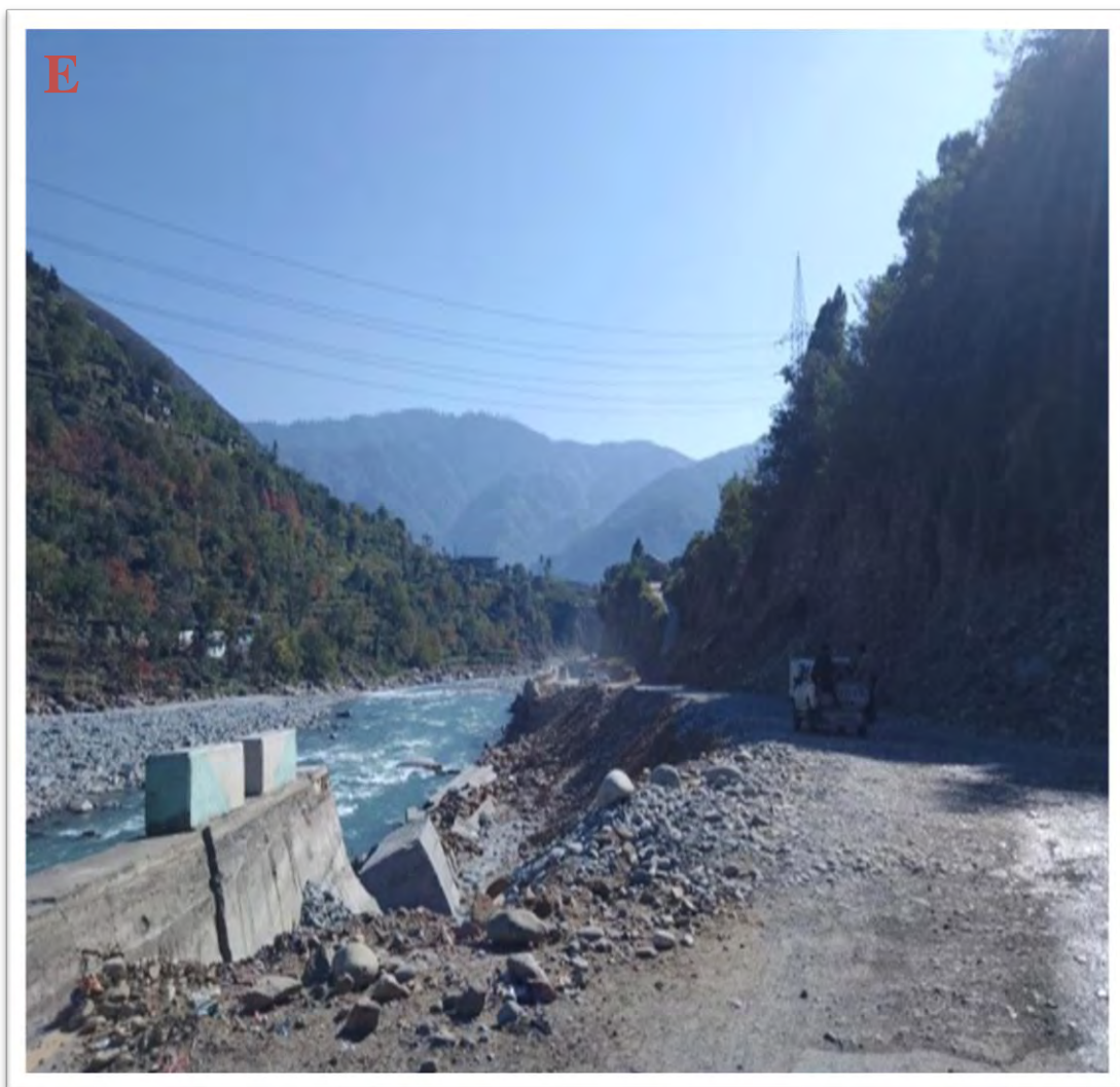
Figure 3.5 E impacts of flood, connecting Bahrain to Mankyal top (Churrai) road completely eroded. The outcrop succession belongs to Kalam group of rocks.
