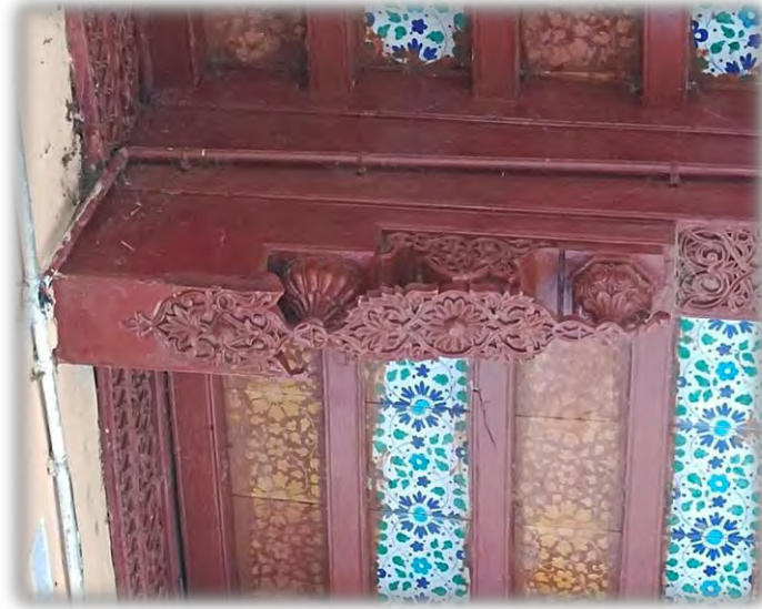
Figure 4.11: Carved Pillar at the roof of Veranda
