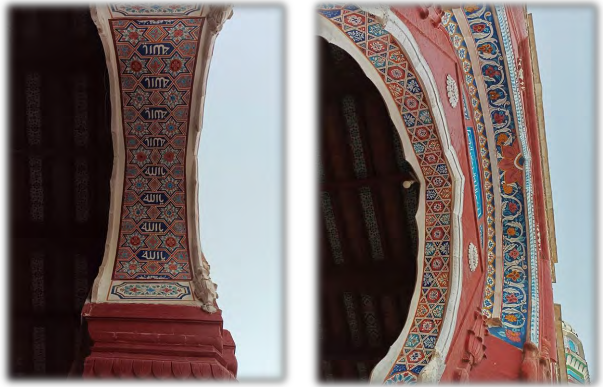
Figure 4.15: Fresco painting and geometrical designs in the interior of multifold Arches
