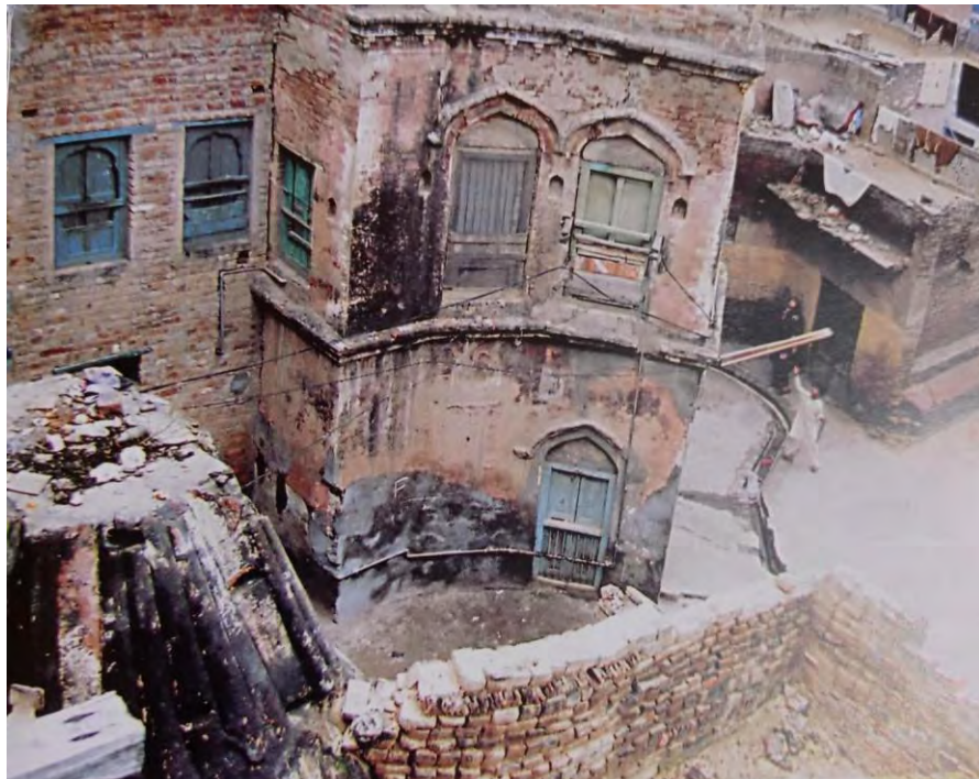
Figure 1: General view of Akbari Baoli
