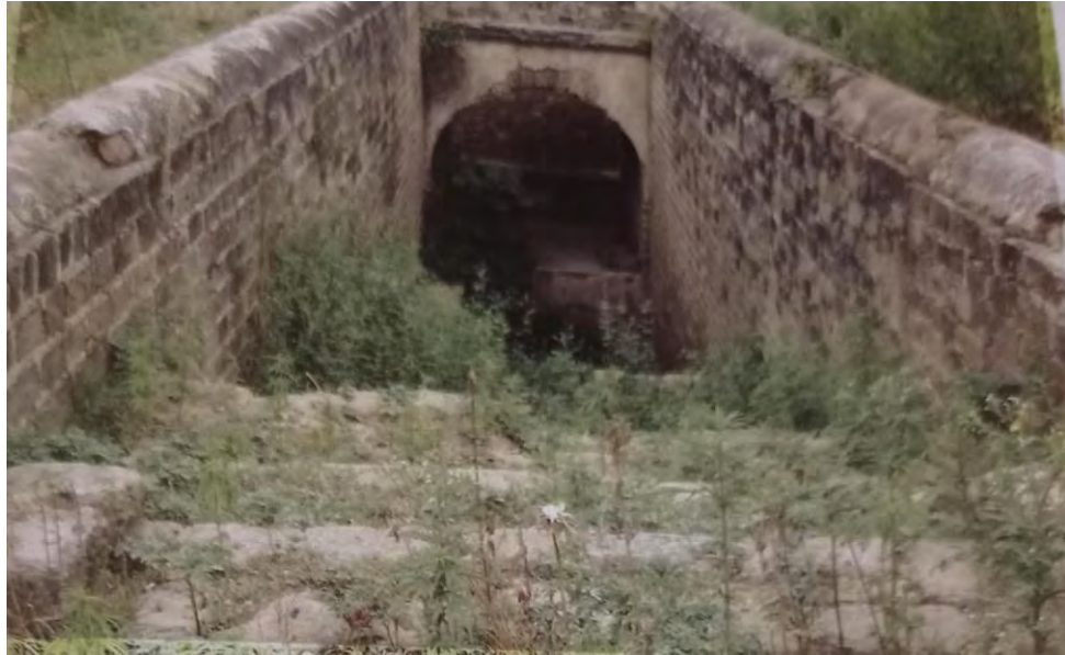
Figure 12: General view of Ghaznabad Baoli, Kalar Sayedan, District Rawalpindi.
