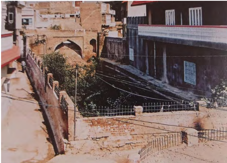
Figure 2: General view (South-East) of Baoli at Khariyan, District Gujrat
