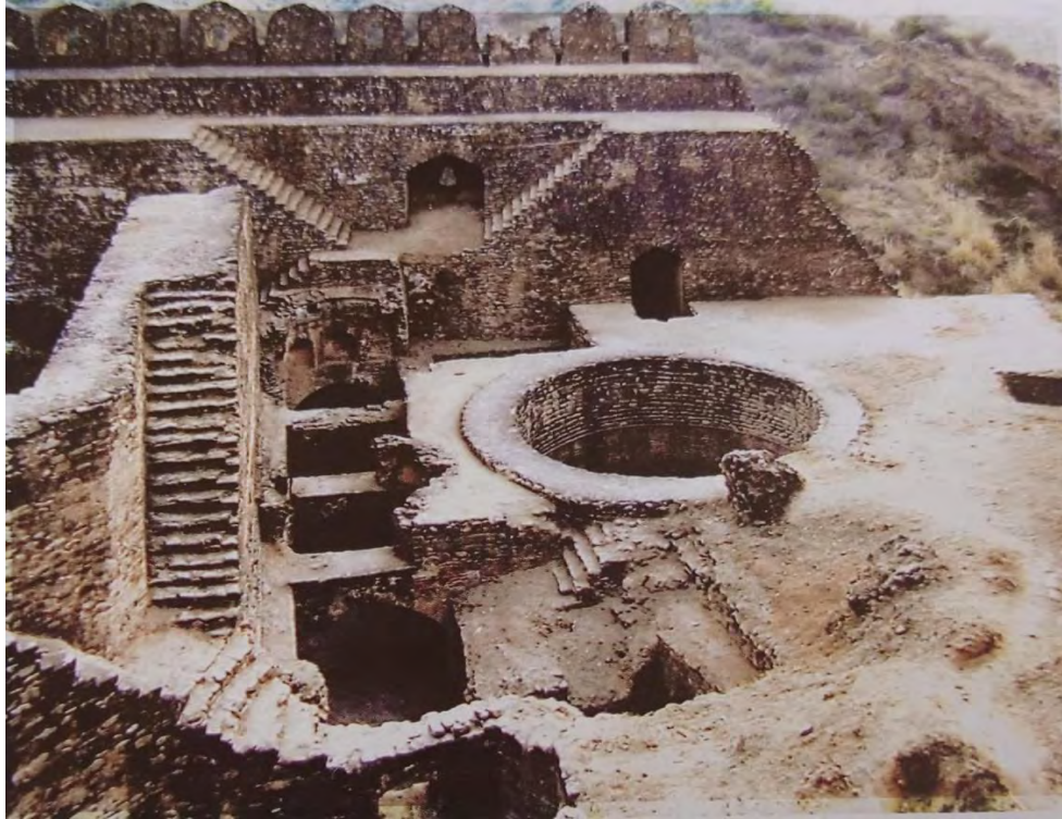
Figure 7: General view of Langar Khan-e- Wali Baoli, Rohtas Fort.
