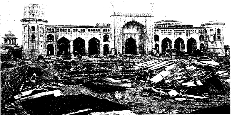
MOSQUE NOW UNDER CONSTRUCTION, BHOPAL
