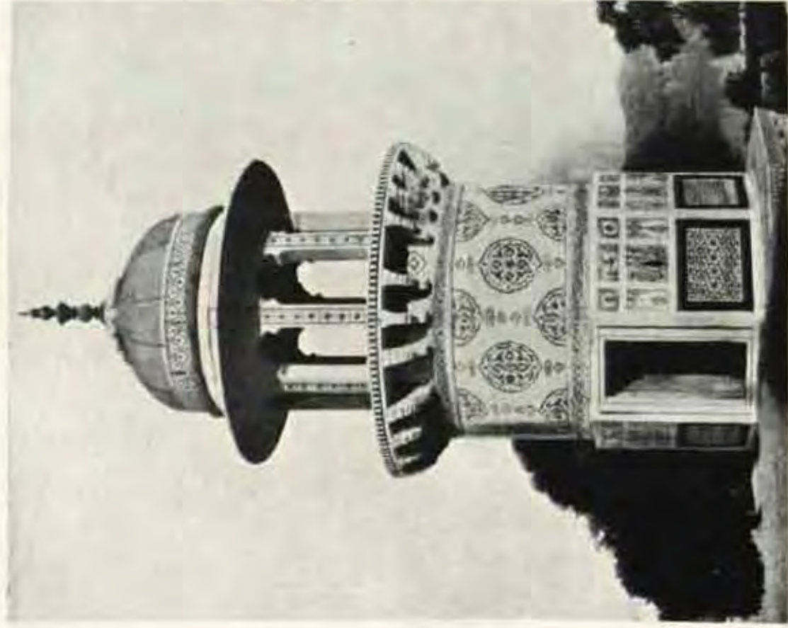
A. Upper part of a corner turret, Itmad-ud-Daula's tomb, Agra, showing pietra dura inlay and marble mosaic.
