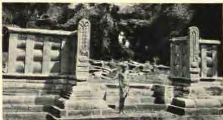
A. Stone railing at Amradhapura, as restored.
