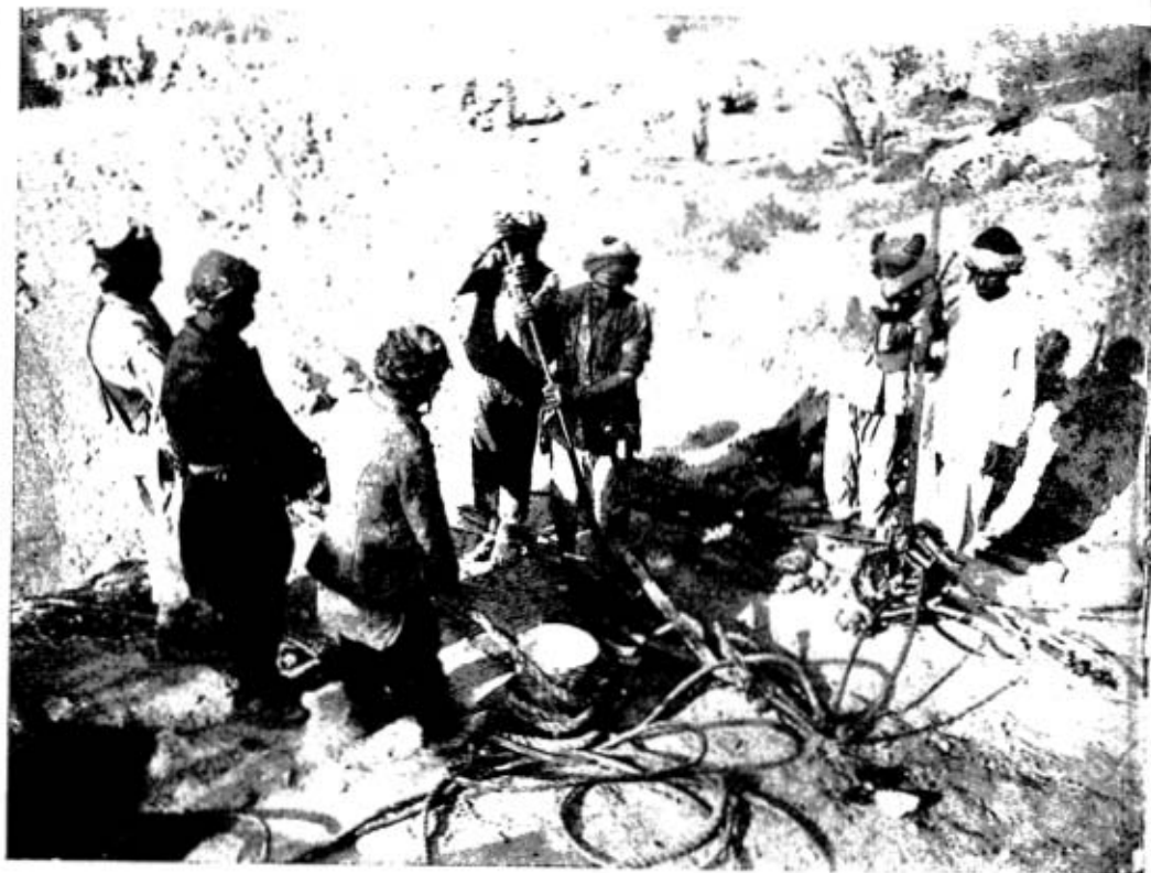
22. Trehwella Winch Operators controlling Bridge Erection
