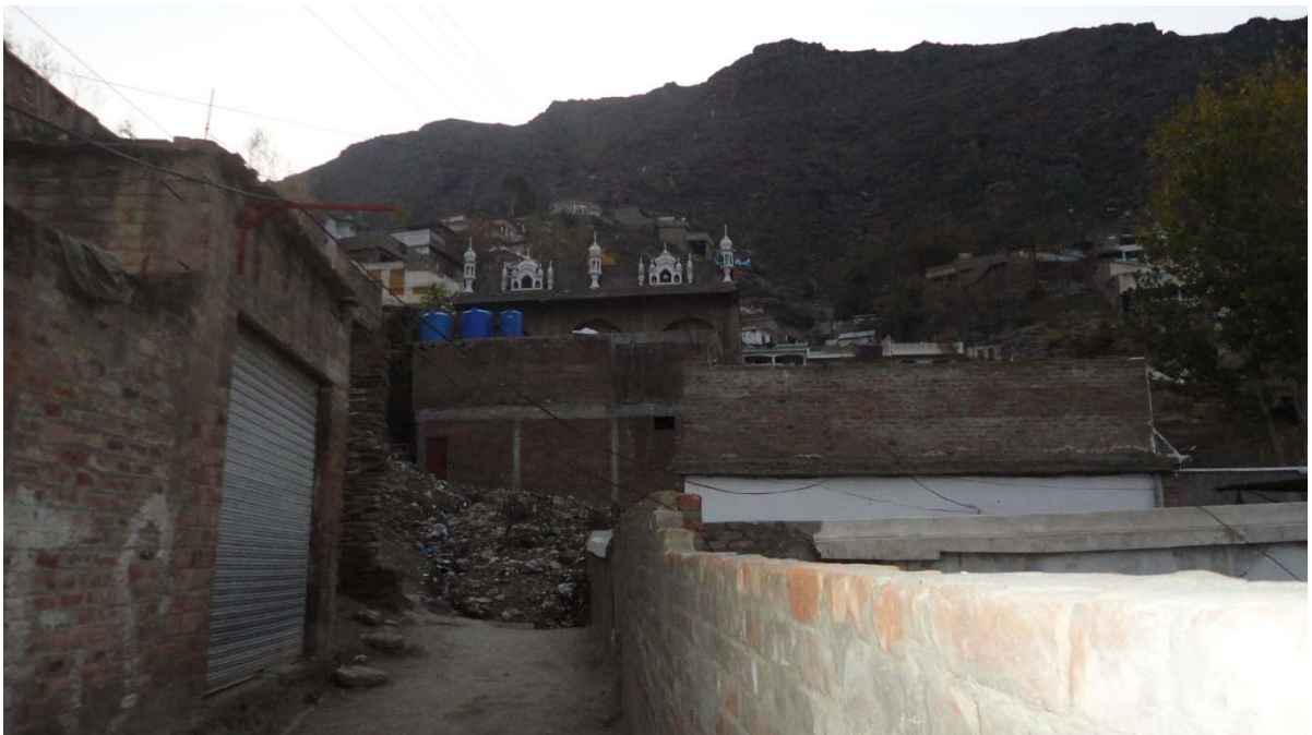
Figure 22: Buildings on the Katelai (Aman-kot) Site
