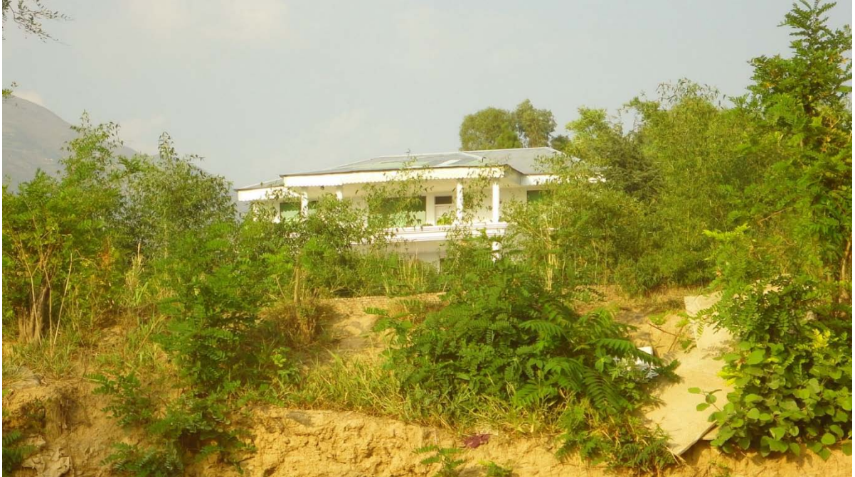
Figure 21: Jampure-dherai, Mangwalthan (Charbagh)
