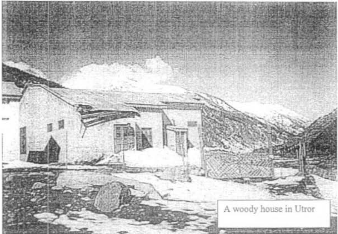
Plate: 2.2. Structure of hoses in village Utror
