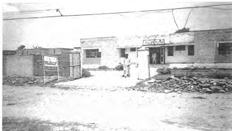
Photograph 1: Basic Health Unit, Jaffer (the boundary wall is being reconstructed)
