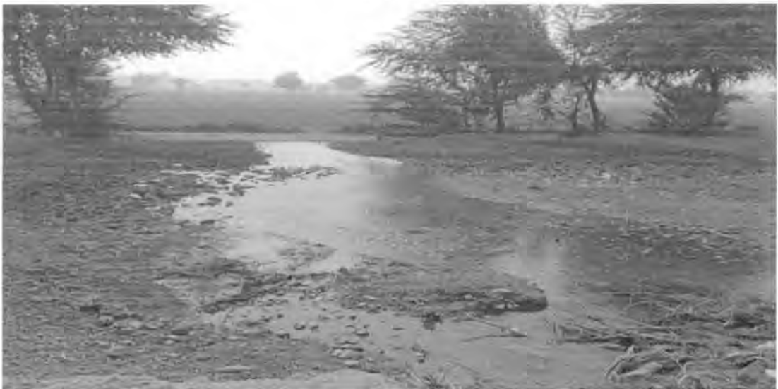
Condition of service road due to over flow of the water from Water Distributary.
