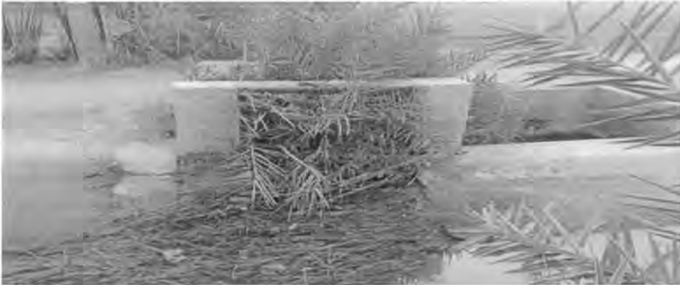
Blockages of Opening of Drainage Channel.
