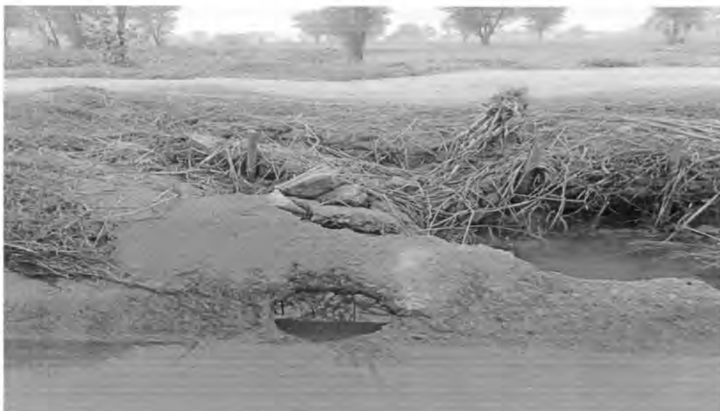
Illustrating the illegal holes in water distributary
