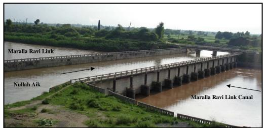
Plate 2.2 Aik crossing over the Maralla Ravi Link canal located near Sahibkay (Site 5). (arrows indicate the direction of flow)
